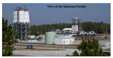
SDF. SPF is permitted as a wastewater treatment facility SCDHEC Regulations per R.61-67. SPF receives and treats the salt solution to produce grout by mixing the LLW liquid stream with cementitious materials (cement, flyash, and slag). A slurry of the components is pumped into the disposal
