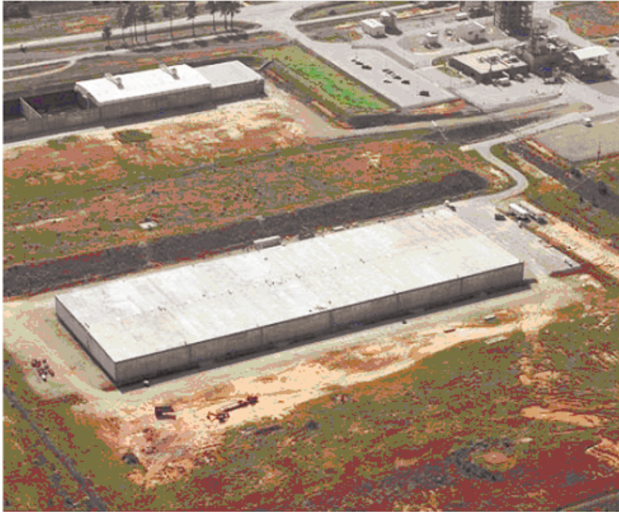
Figure 4 Photograph of Existing SDF Vault 4
