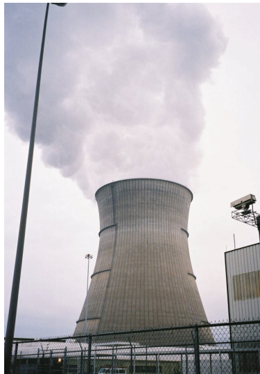
Natural Draft Cooling Tower
