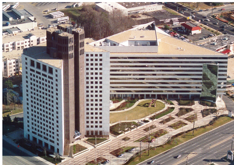
NRC Offices in Rockville, Maryland
