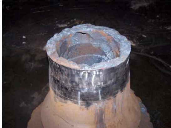
Surge nozzle after flapping and plug removal
