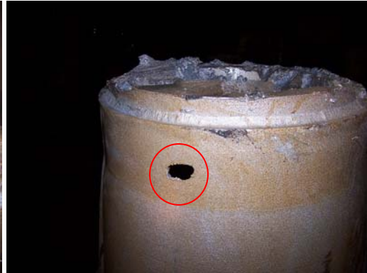
Flame cut hole in the DM weld
