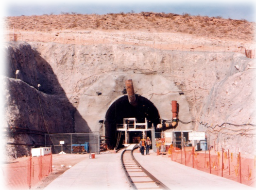
Entrance Tunnel at Yucca Mountain
