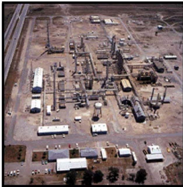
Figure 3- 8 DCP Midstream Linam Ranch Plant Southeast of the IIFP Facility
