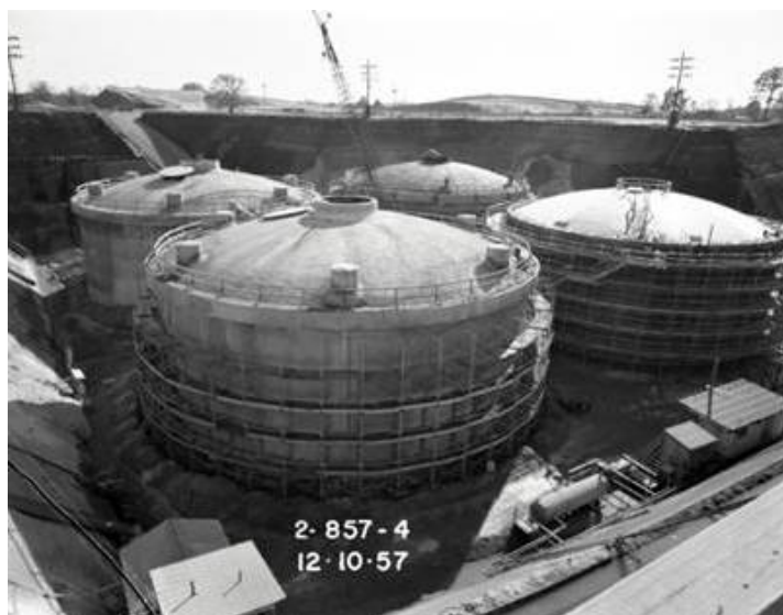
Figure 2.1-47: Typical Type IV Waste Tank Domes and Risers During Construction
