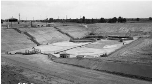
Figure 2.1-30: Type I Waste Tank Basemat Construction
