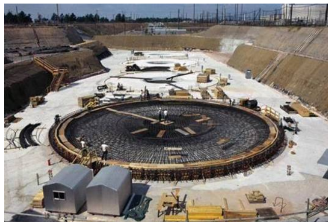
Figure 2.1-37: Typical Type III/IIIA Waste Tank Basemat Construction
