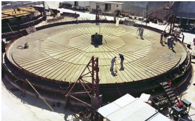
Figure 2.1-39: Typical Type III/IIIA Waste Tank Radial Air Grooves
