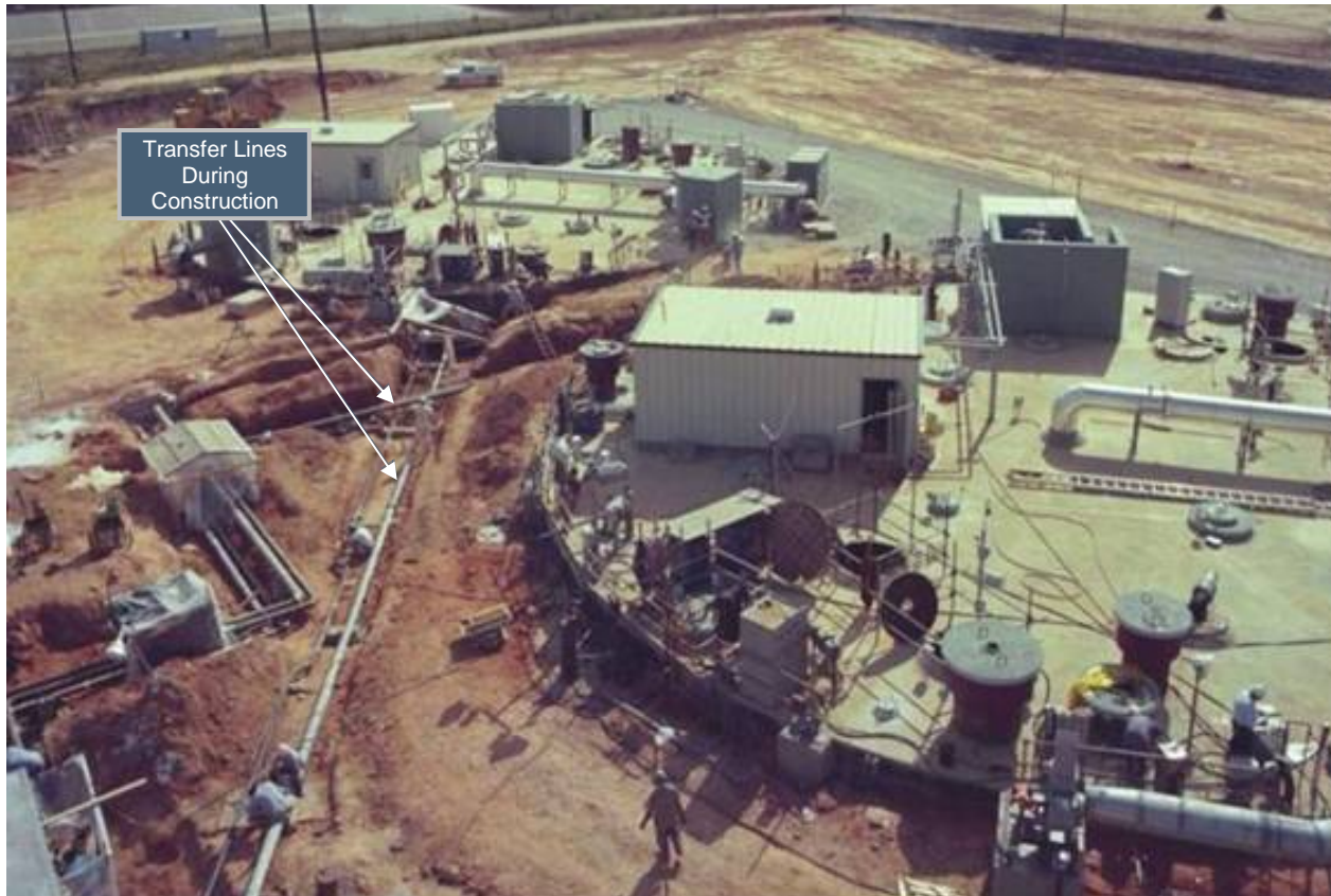
Figure 2.1-49: Typical Waste Tank Transfer Line During Construction
