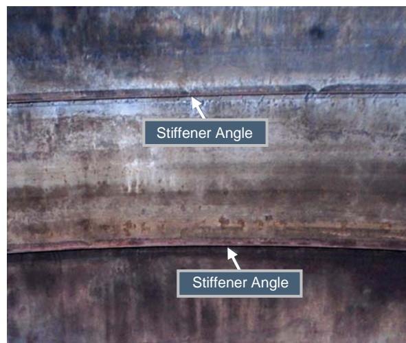
Figure 2.1-45: Typical Type IV Waste Tank Stiffener Angles
