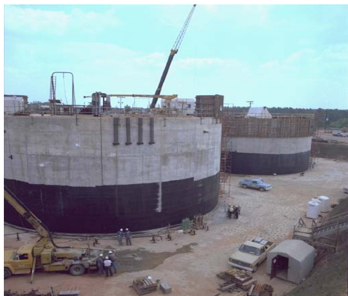
Figure A.2-1: Waste Tanks Under Construction
