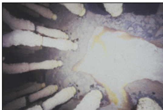
Salt waste is dissolved in the liquid portion of the waste. It can be in normal solution as Supernate (top picture) or, after evaporation, as salt cake (bottom picture) or concentrated supernate. The pipes in all the pictures are cooling coils.
