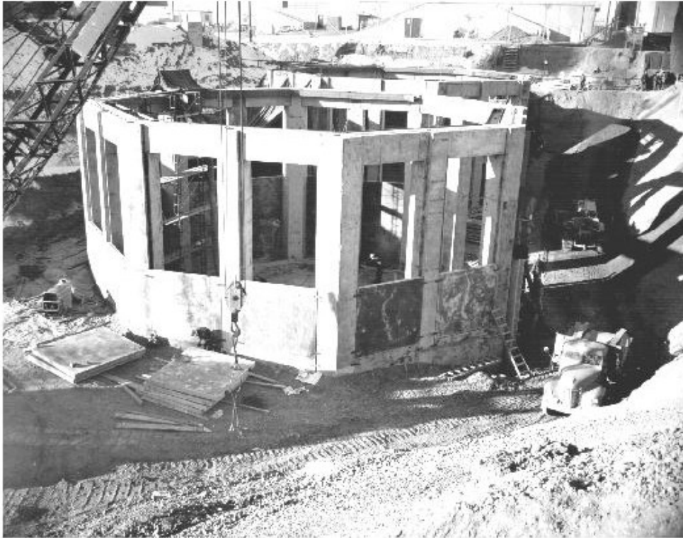
Figure 1-5. Pillar and panel octagonal vault for Tank WM-183.
