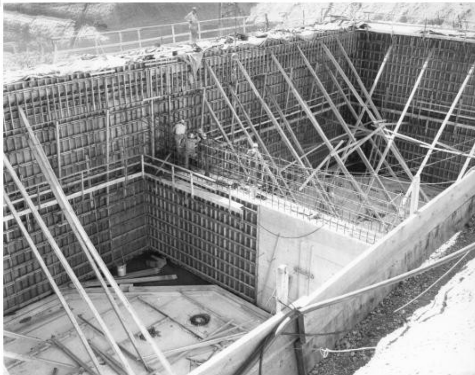
Figure 1-6. Monolithic square vault for Tank WM-190.
