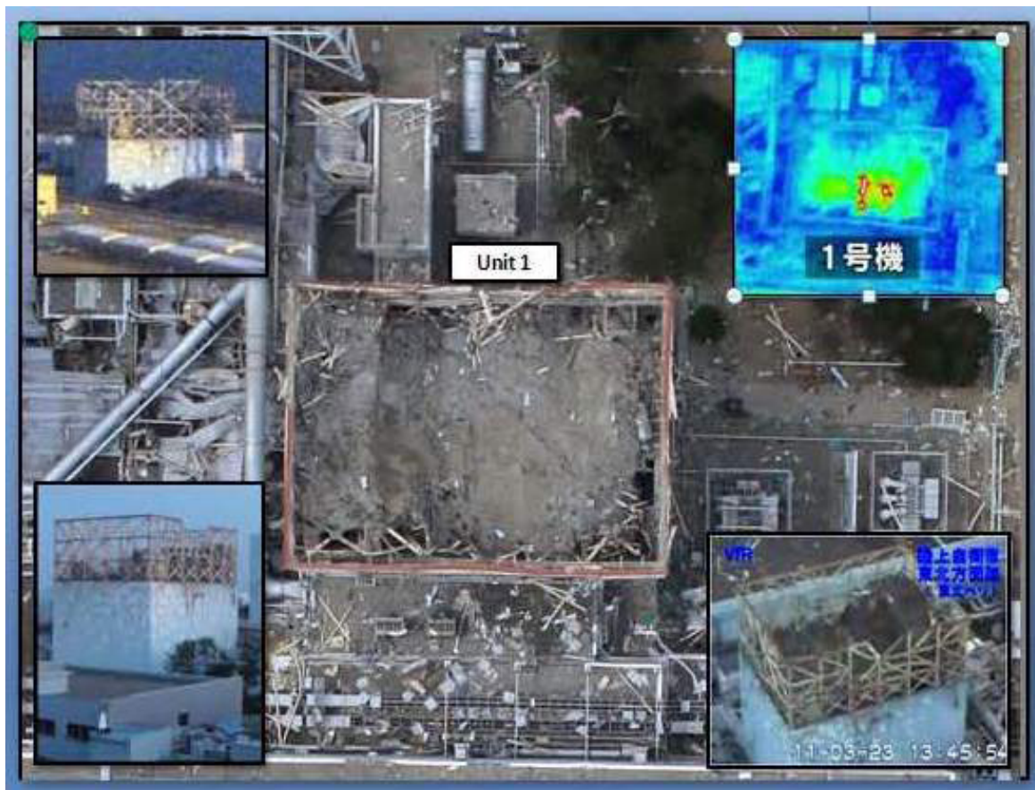
Figure 3: Damage to Unit 1
