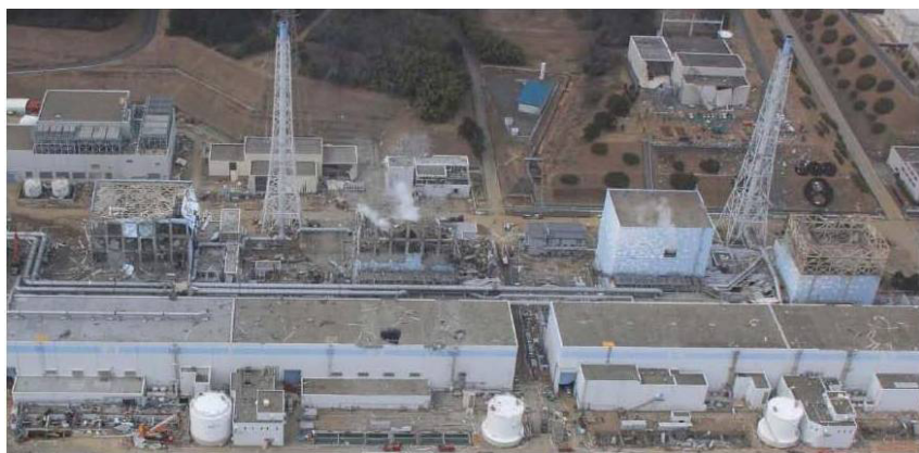
Figure 7: Fukushima Dai-ichi Units 1–4 following explosions
