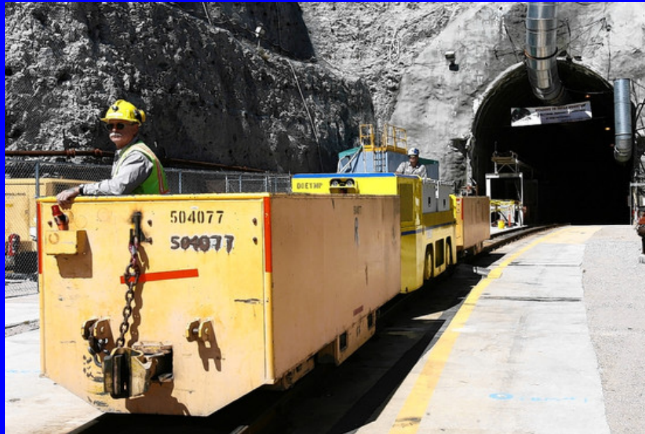
Yucca Mountain Tunnel Entrance
