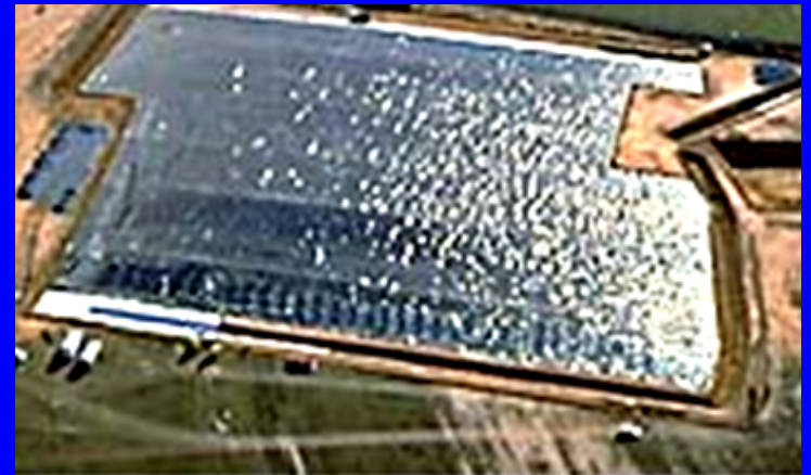
Above: engineered cap/cover over filled “trench” Barnwell
