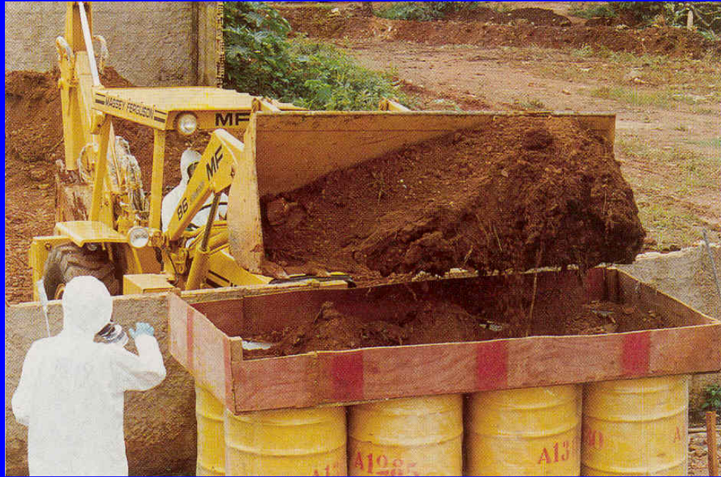
Filling drums with contaminated soil
