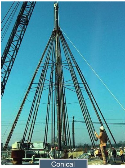
Figure 2.1-40: Typical Type III Waste Tank Deployable Cooling Coils
