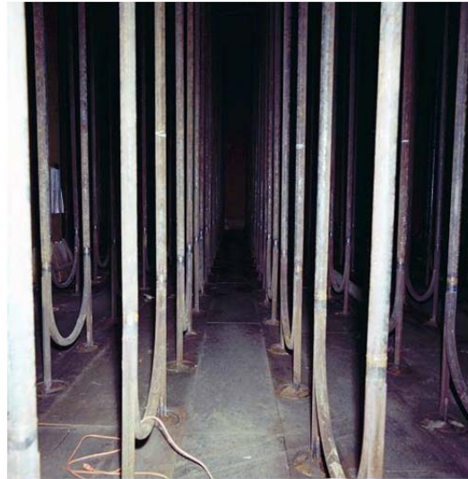
Figure 2.1-41: Typical Type IIIA Waste Tank Cooling Coils During Construction
