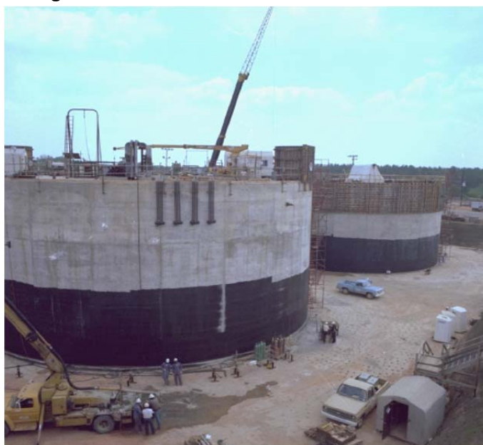
Figure A.2-1: Waste Tanks Under Construction
