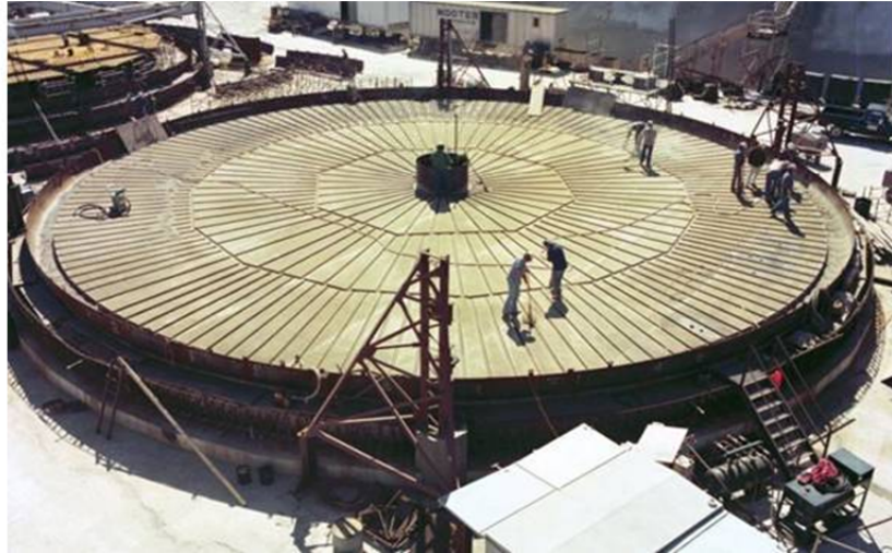
Figure 2.1-39: Typical Type III/III A Waste Tank Radial Air Grooves
