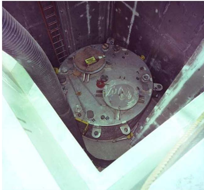
Figure 2.1-52: Typical Pump Tank Top View During Construction
