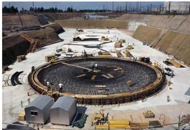
Figure 2.1-37: Typical Type III/IIIA Waste Tank Basemat Construction
