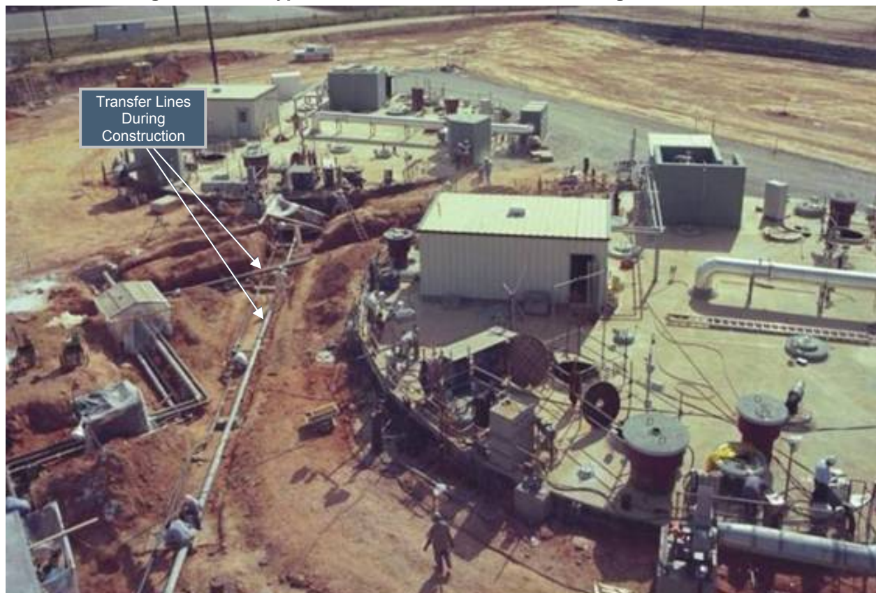
Figure 2.1-50: Typical Waste Tank Transfer Line During Construction
