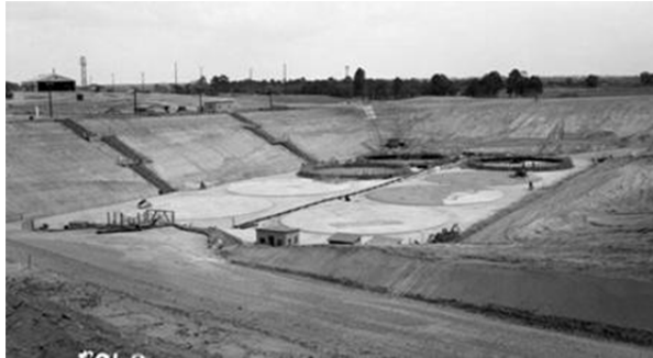
Figure 2.1-30: Type I Waste Tank Basemat Construction
