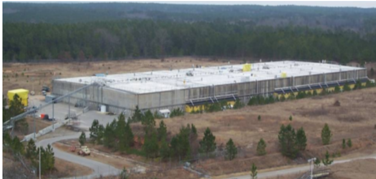
Figure 1.3-2: Vault 4 at the SDF (SRR-CWDA-2010-00013)
