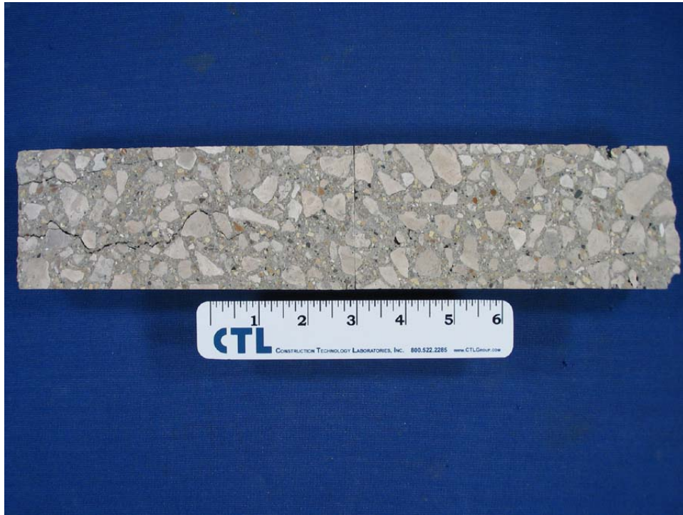
Fig. 4 Lapped cross-section of the core sample showing the general appearance and condition of the concrete. Top surface is to the left.
