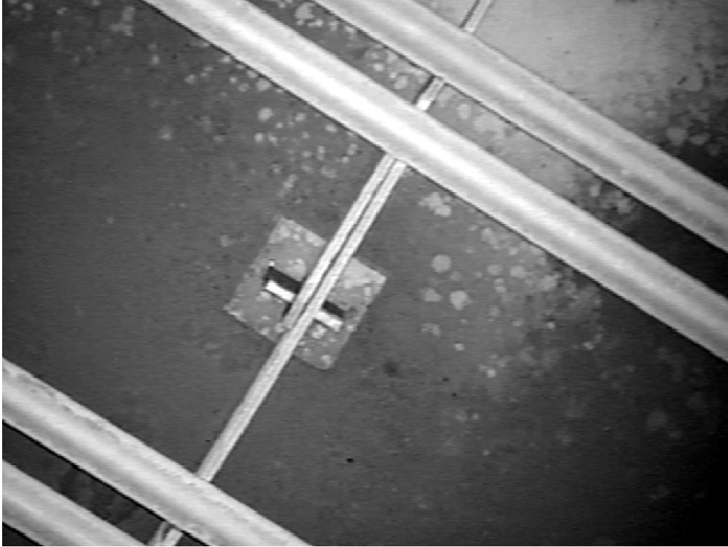
Figure A-4. TFF Tank WM-183 post-decontamination interior.
