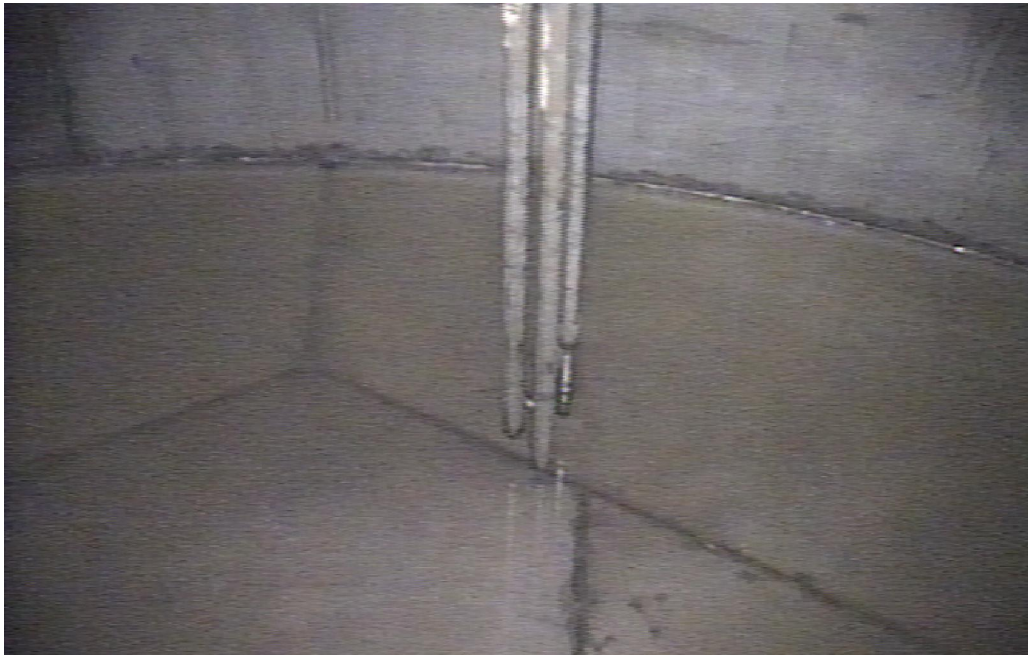
Figure A-5. TFF Tank WM-184 post-decontamination interior.
