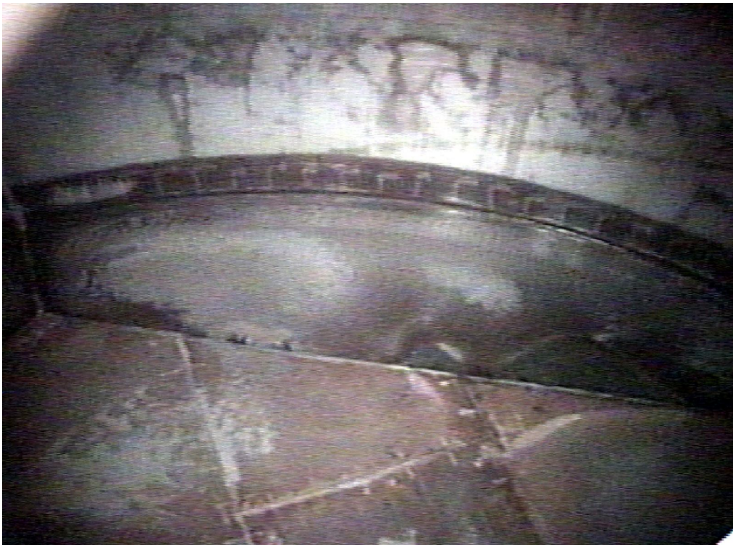
Figure A-7. TFF Tank WM-186 post-decontamination interior.
