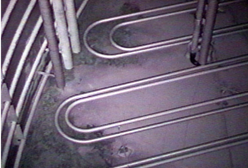
Figure A-6. TFF Tank WM-185 post-decontamination interior.
