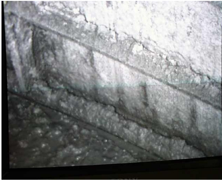
Figure 11. Photographs of the interior of TFF Tank WM-183 before tank cleaning.
