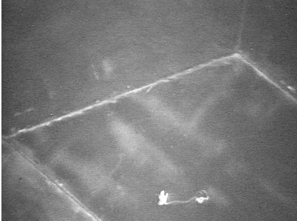
Figure A-2. TFF Tank WM-181 post-decontamination interior.
