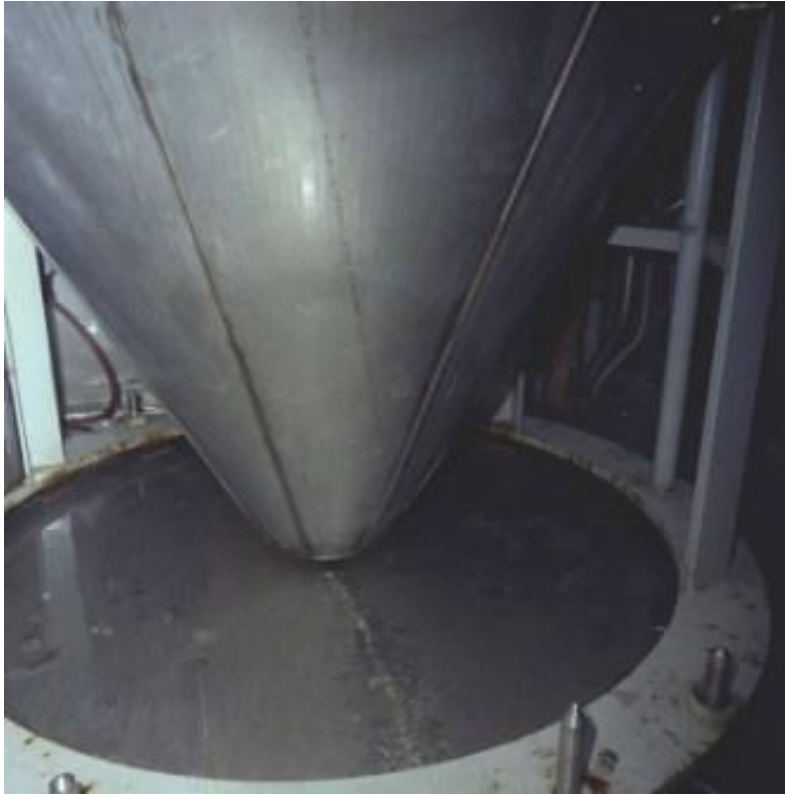
Figure 3.2-70: View of the Bottom of the 242-25H Evaporator Vessel
