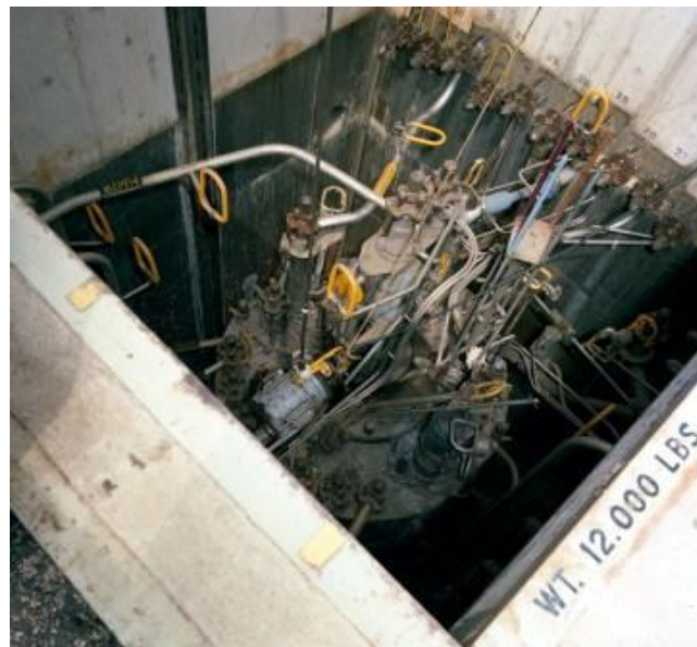
Figure 3.2-63: Concentrate Transfer System PP and Pump Tank
