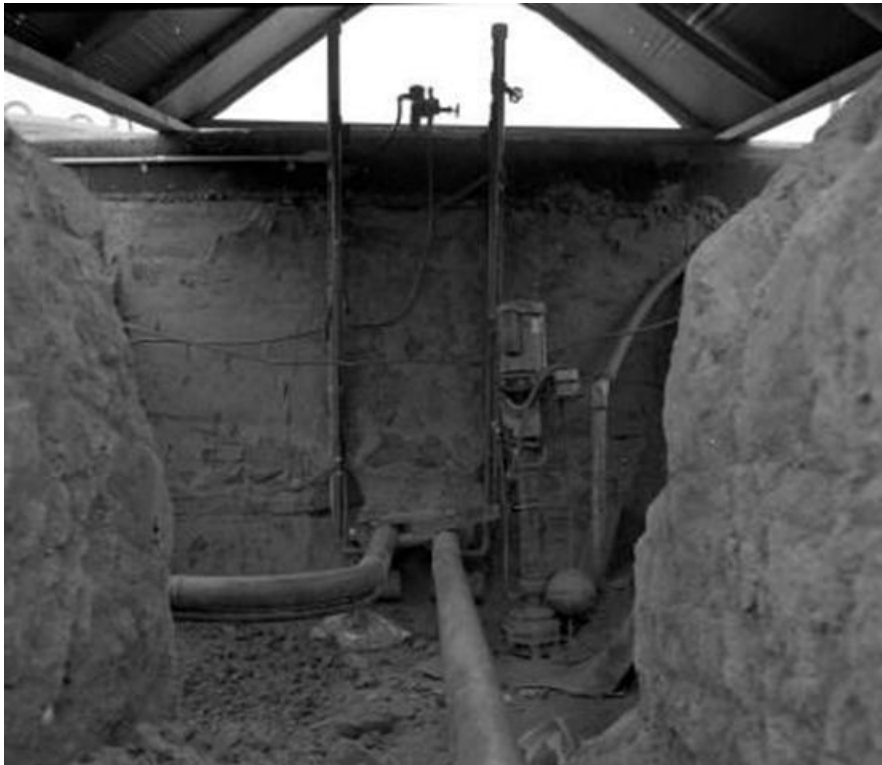
Figure 3.2-55: HTF Transfer Line Construction at Tank 30H
