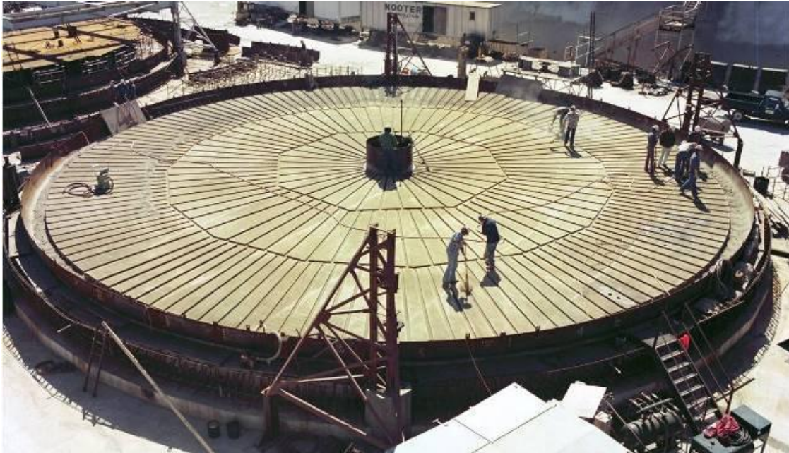
Figure 3.2-33: Typical Type IIIA Tank Primary and Secondary Liner - Early Construction
