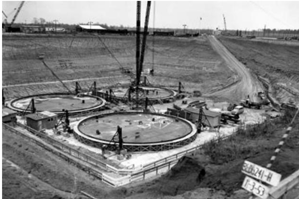
Figure 3.2-5: Typical Basemat Construction for Type I Tanks
