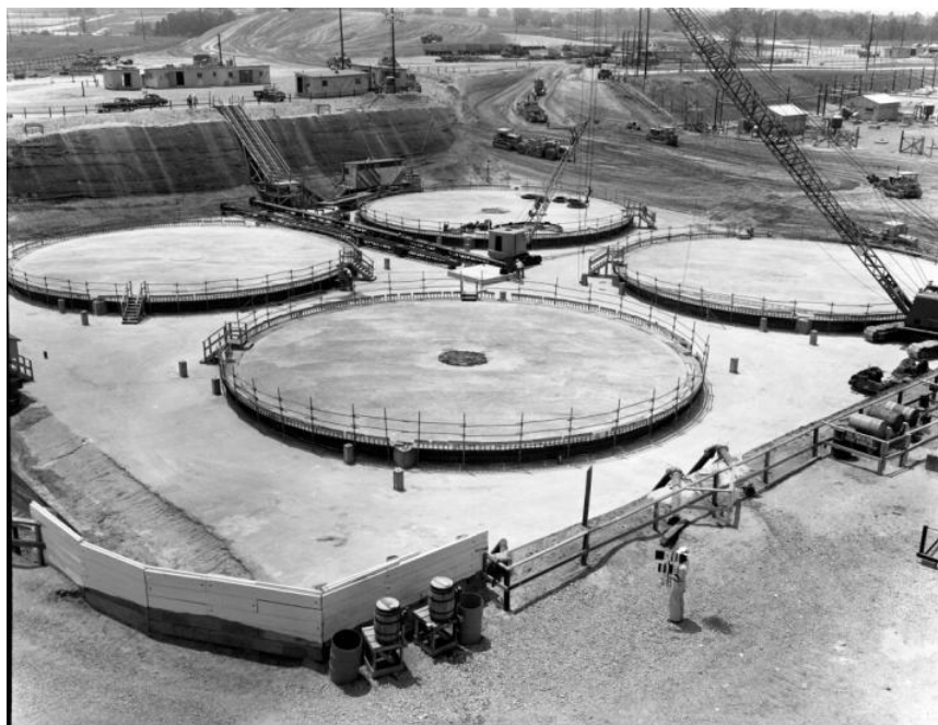
Figure 4.2-25: Working Slab for Tanks 13 through 16
