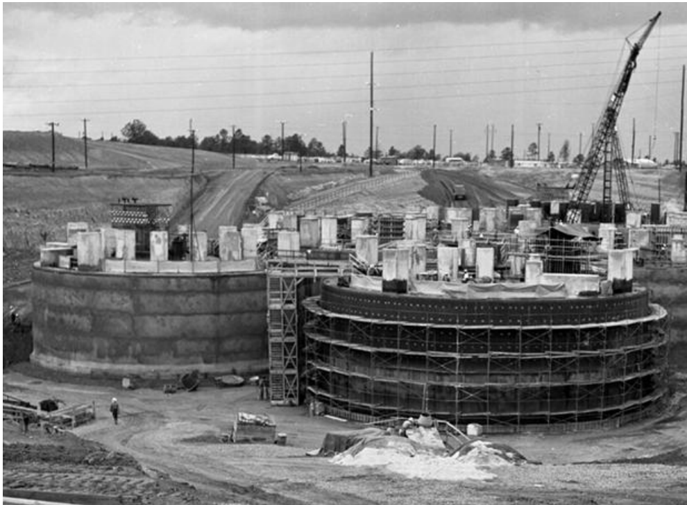
Figure 3.2-10: Typical Riser Construction for Type I Tanks
