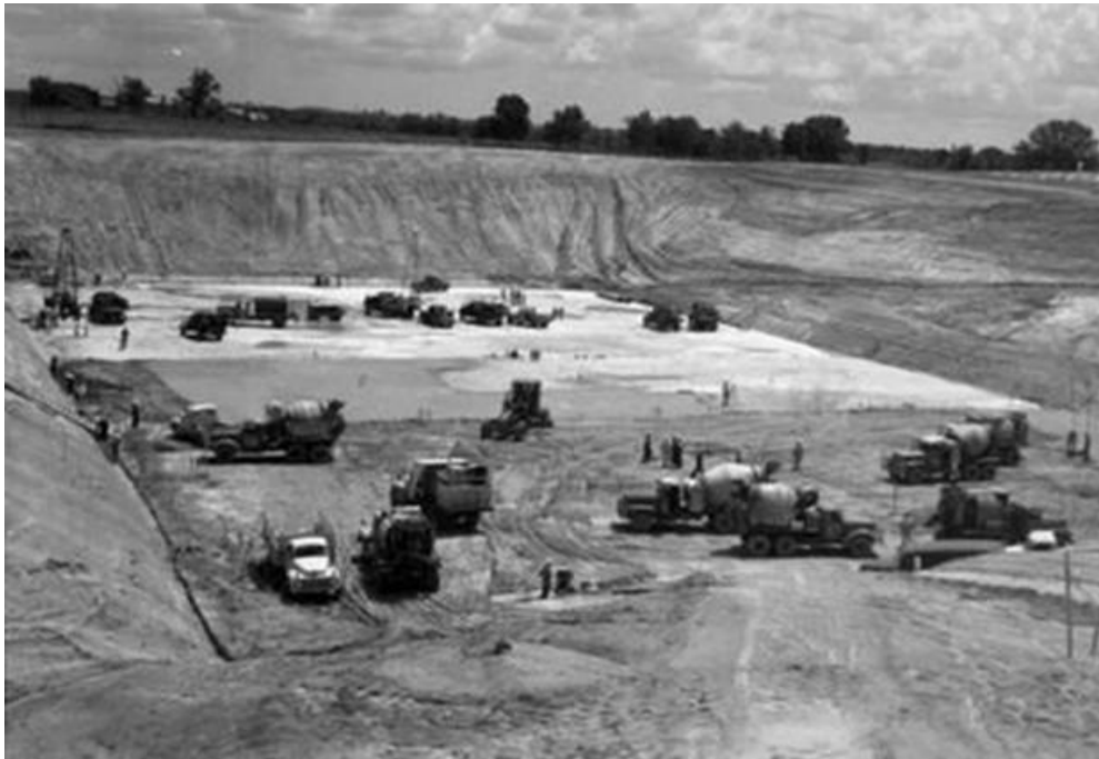
Figure 3.2-5: Typical Basemat Construction for Type I Tanks
