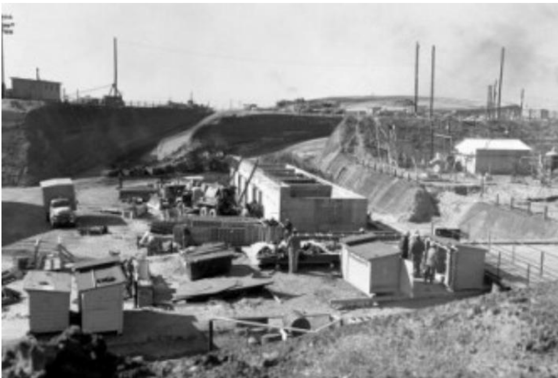
Figure 3.2-60: Construction of Typical HTF PP
