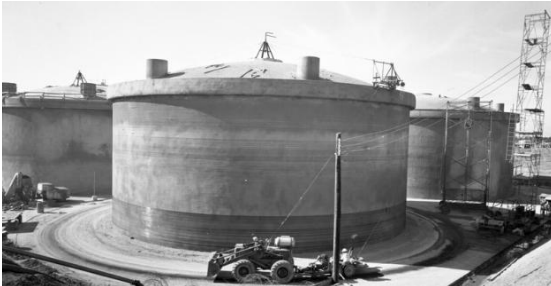
Figure 3.2-50: Type IV Tank Concrete Vault Construction
