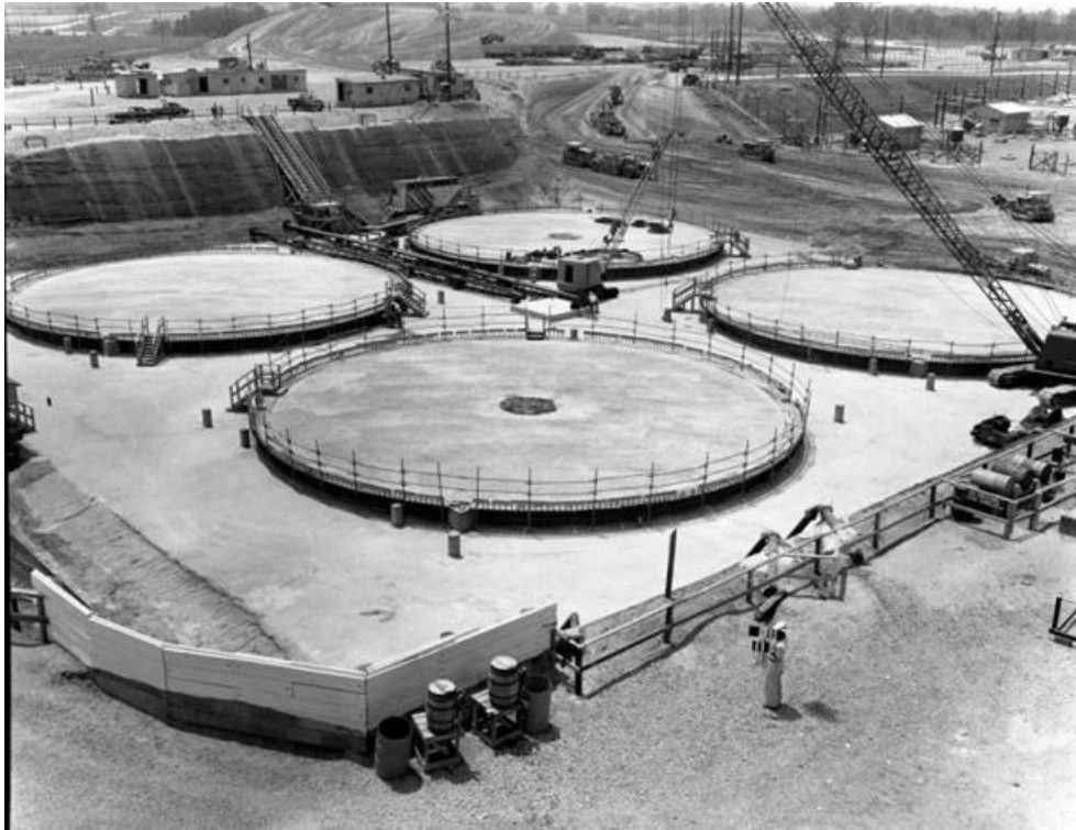
Figure 3.2-17: Type II Tank Working Slab and Basemat
