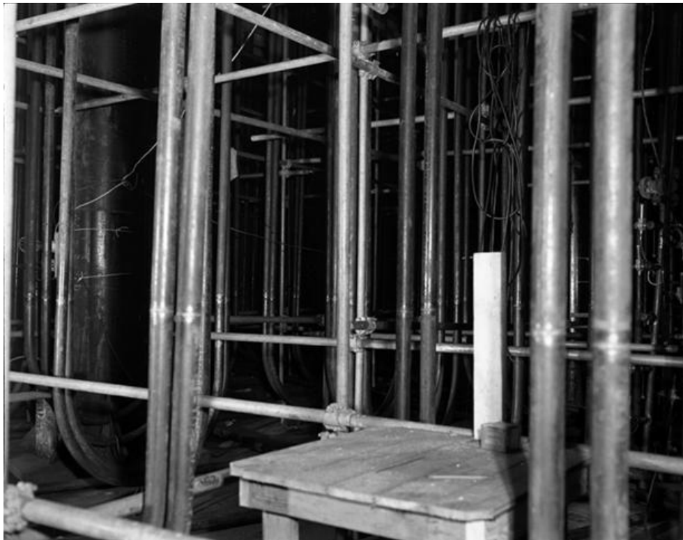
Figure 3.2-14: Type I Tank Cooling Coils - Construction Phase
