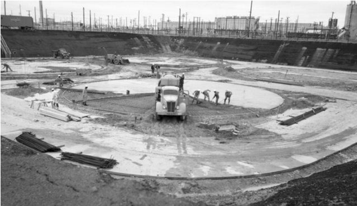
Figure 3.2-47: Type IV Tank Basemat Showing Geometry of Drainage Channels
