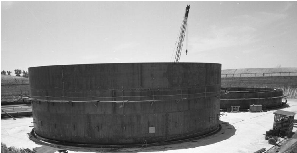
Figure 3.2-48: Type IV Tank Primary Liner Construction
