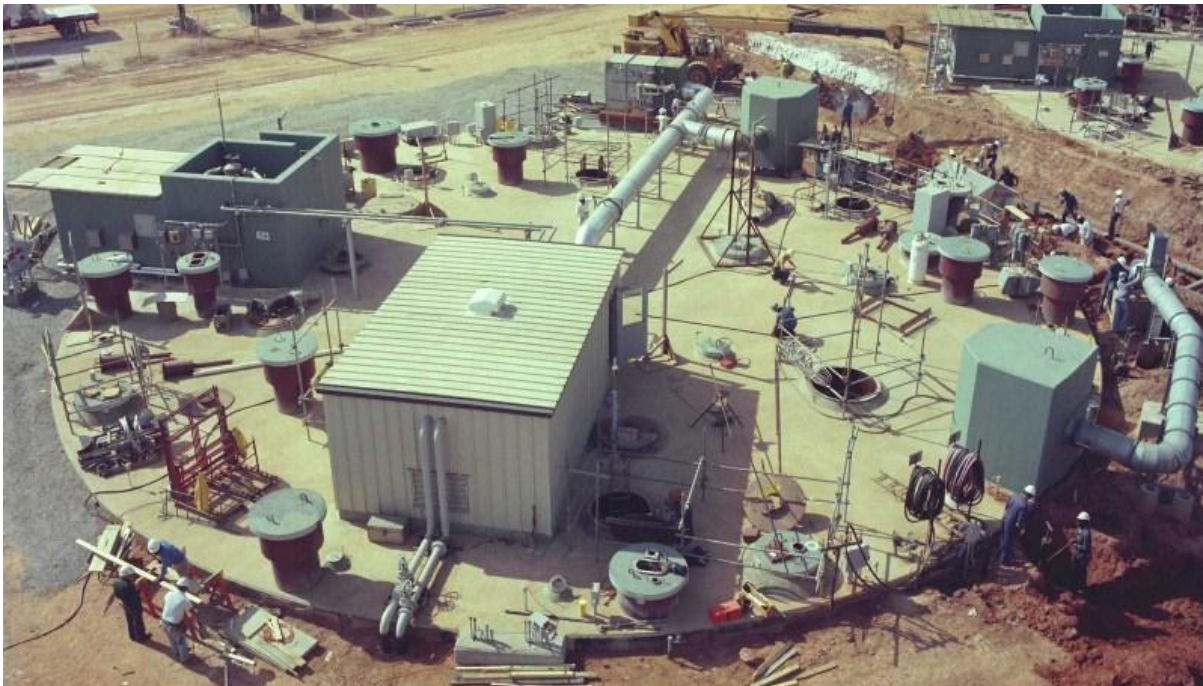
Figure 3.2-44: Typical Type III and IIIA Tank - Backfill Complete
