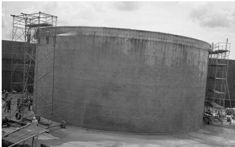
Figure 3.2-51: Type IV Tank Vault Wall Shotcrete Application
