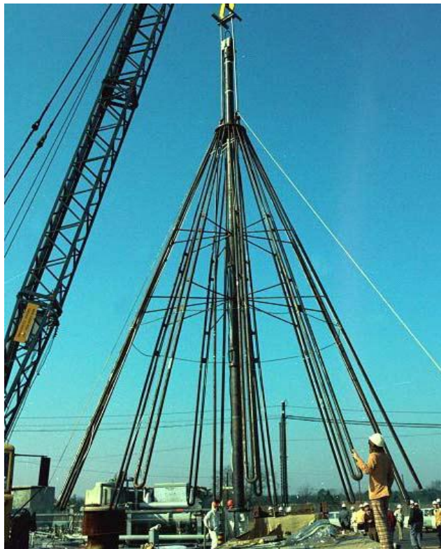
Figure 3.2-42: Typical Conical (Umbrella) Type of Deployable Cooling Coil
