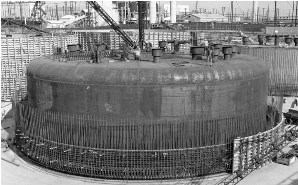
Figure 3.2-21: Type II Tank - Early Stage of Vault Construction
