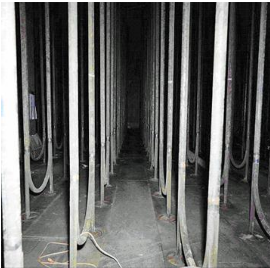
Figure 3.2-43: Cooling Coils in a Type IIIA Tank
