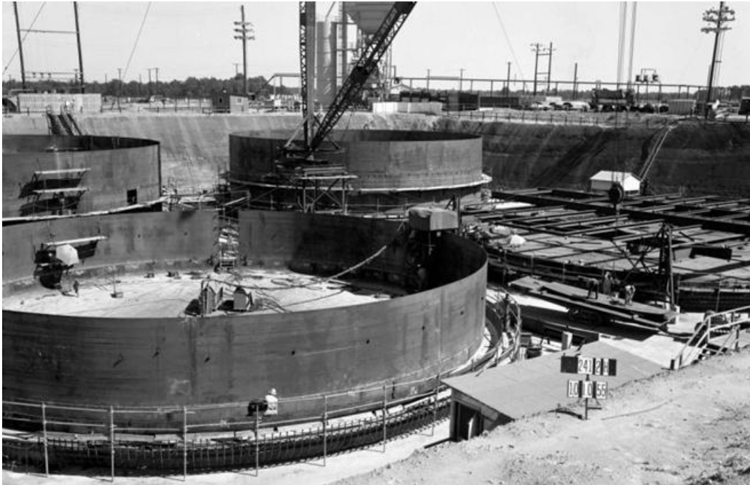
Figure 3.2-20: Type II Tank Early Construction of Primary and Secondary Liner
