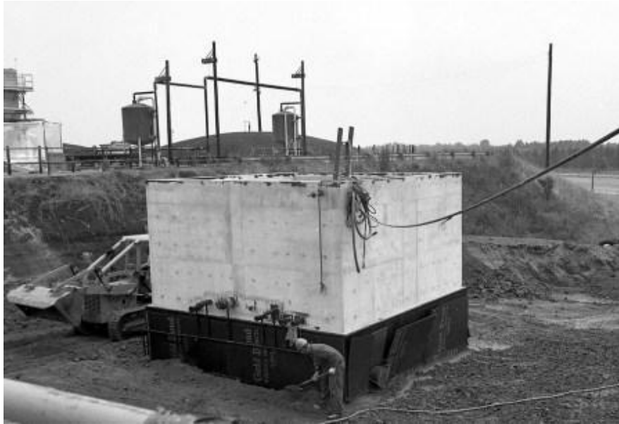
Figure 3.2-62: Construction of HTF CTS PP Building 242-3H (Old)
