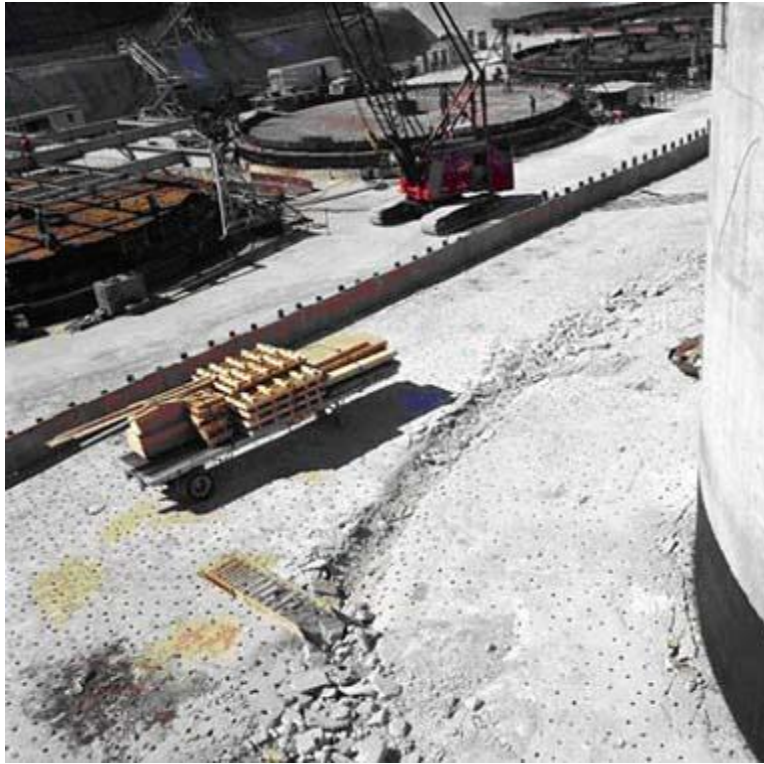
Figure 3.2-30: Drilled Working Slab of a Type IIIA Tank
