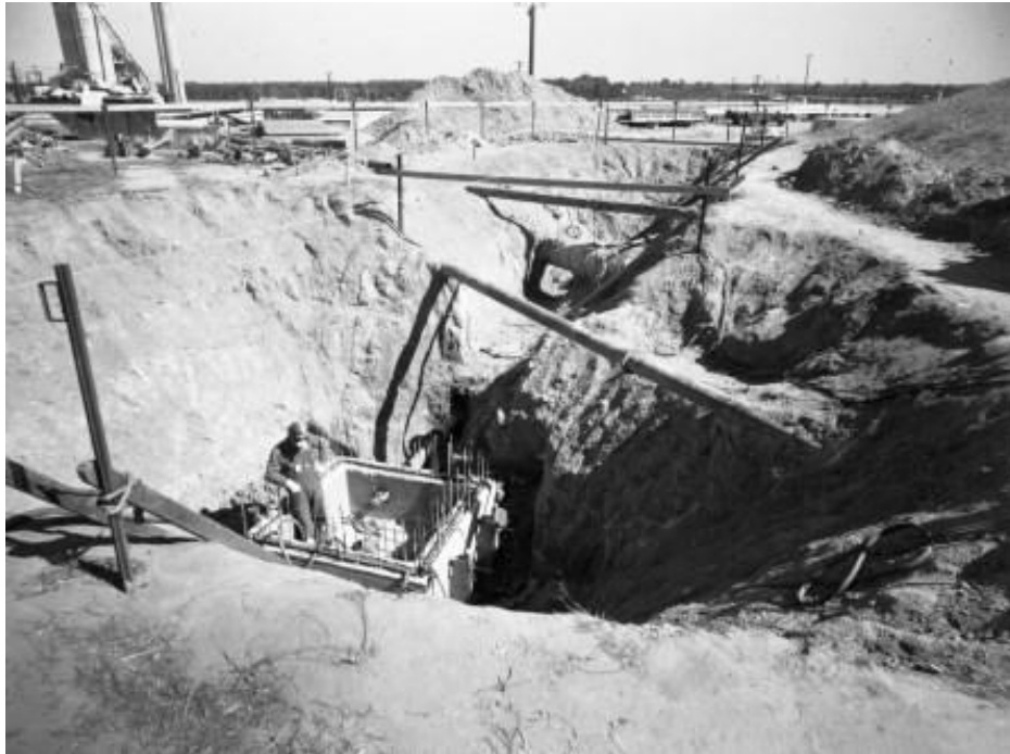
Figure 3.2-73: HDB-3 during Construction Phase
