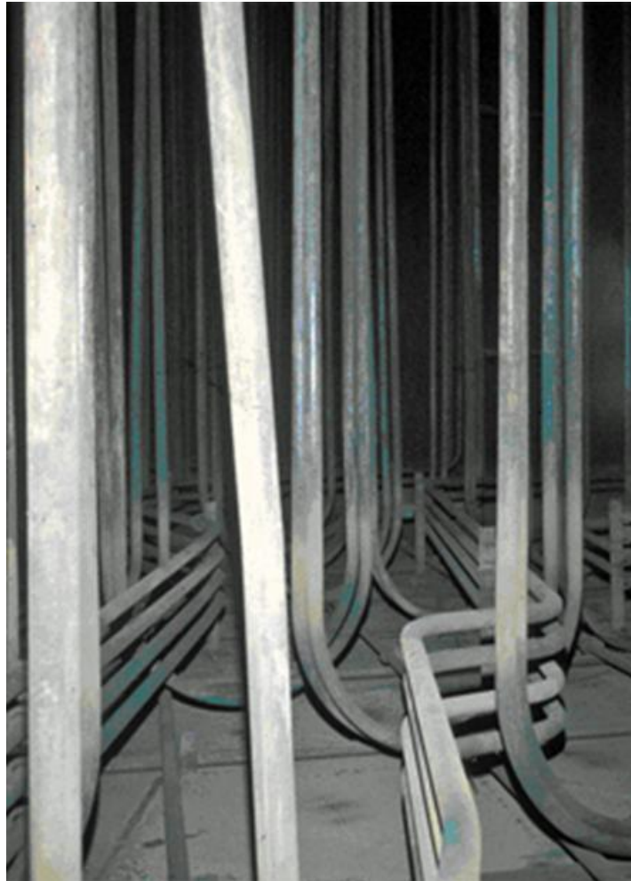
Figure 3.2-25: Type II Tank Cooling Coils
