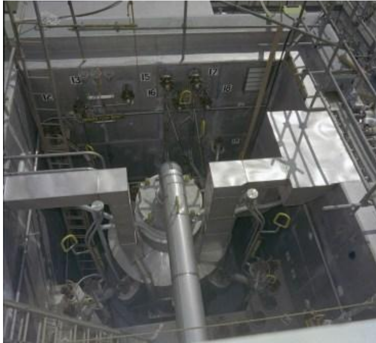
Figure 3.2-69: 242-25H Evaporator Vessel and Cell Top View
