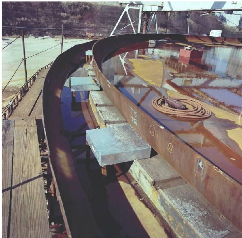
Figure 3.2-33: Typical Type IIIA Tank Primary and Secondary Liner - Early Construction
