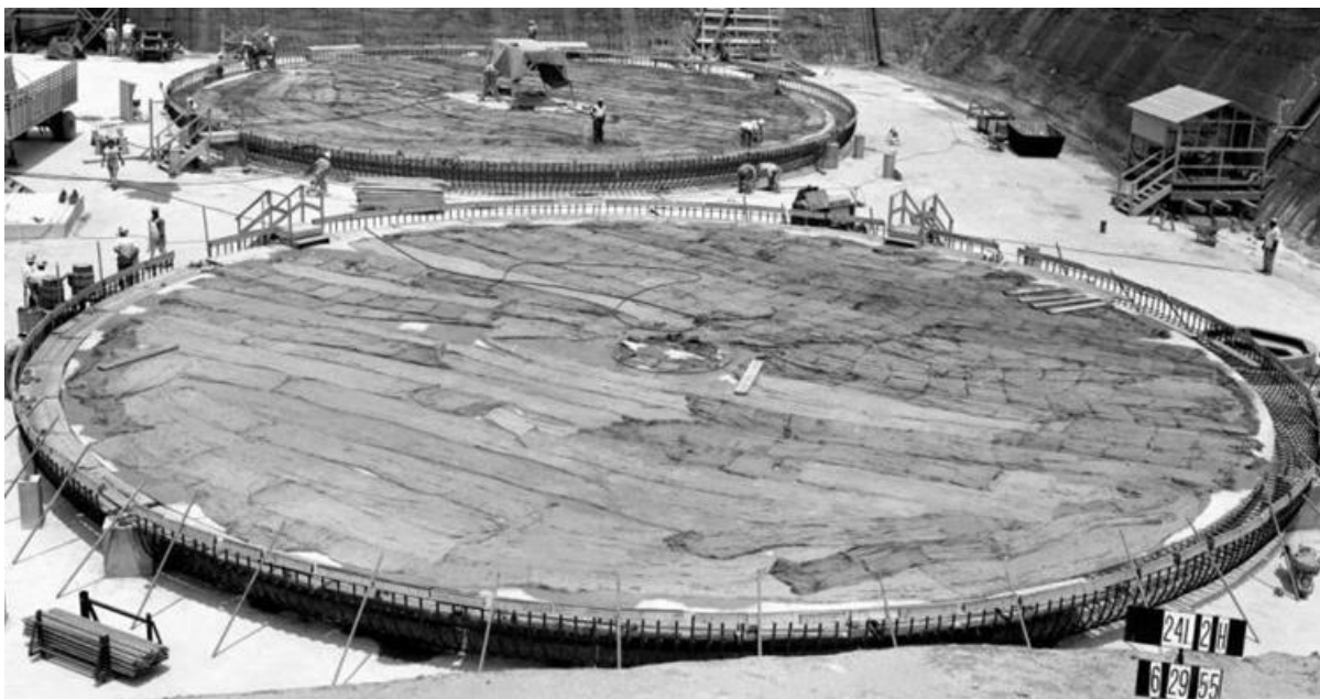
Figure 3.2-19: Lower Sand Pad Installation over the Basemat
