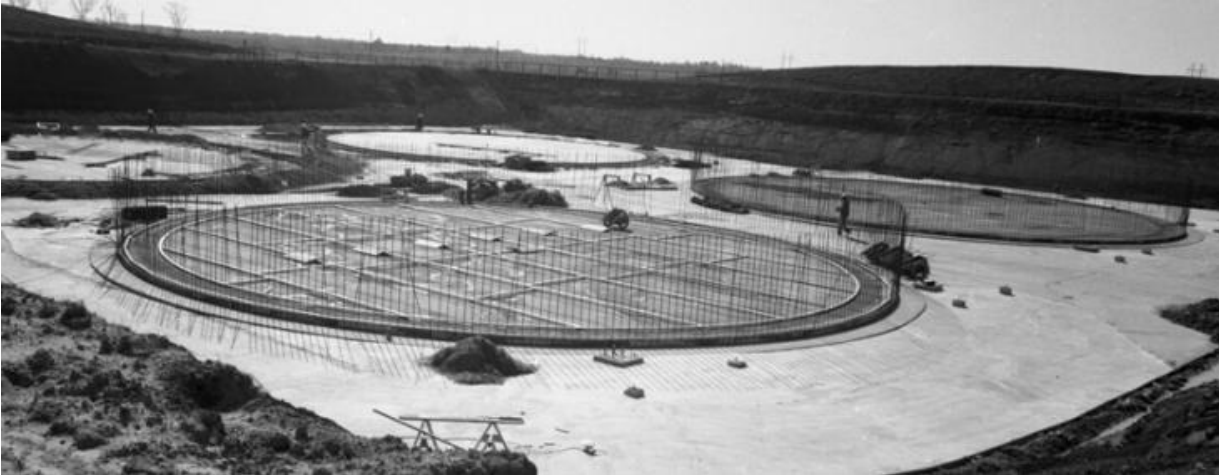
Figure 3.2-47: Type IV Tank Basemat Showing Geometry of Drainage Channels
