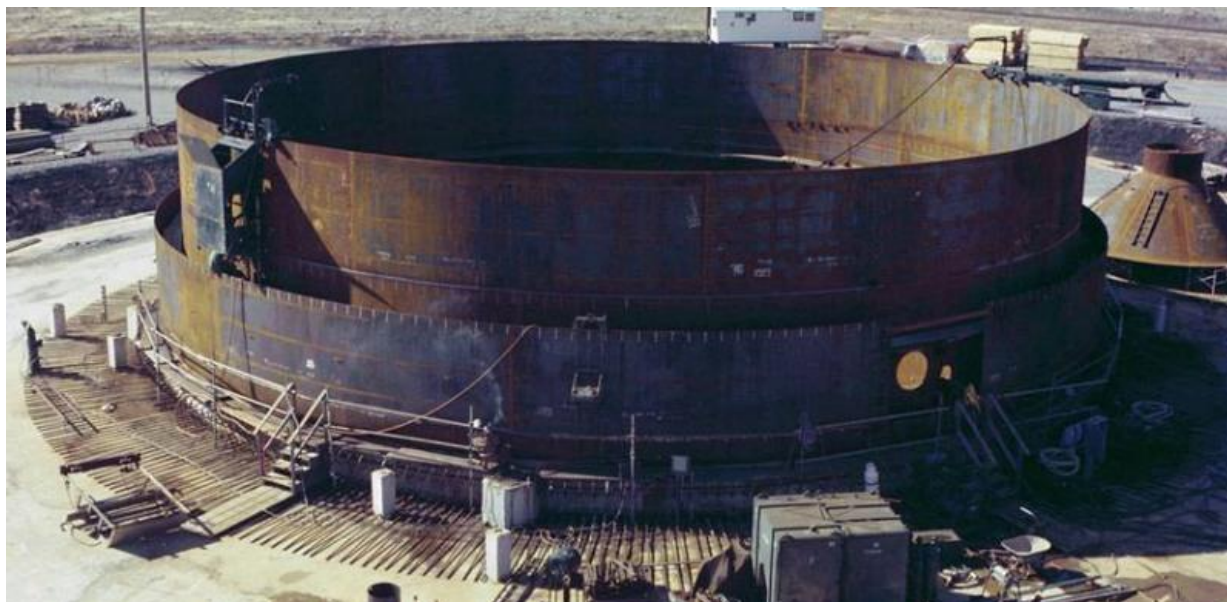
Figure 3.2-34: Typical Type IIIA Tank Primary and Secondary Liner - Partial Construction
