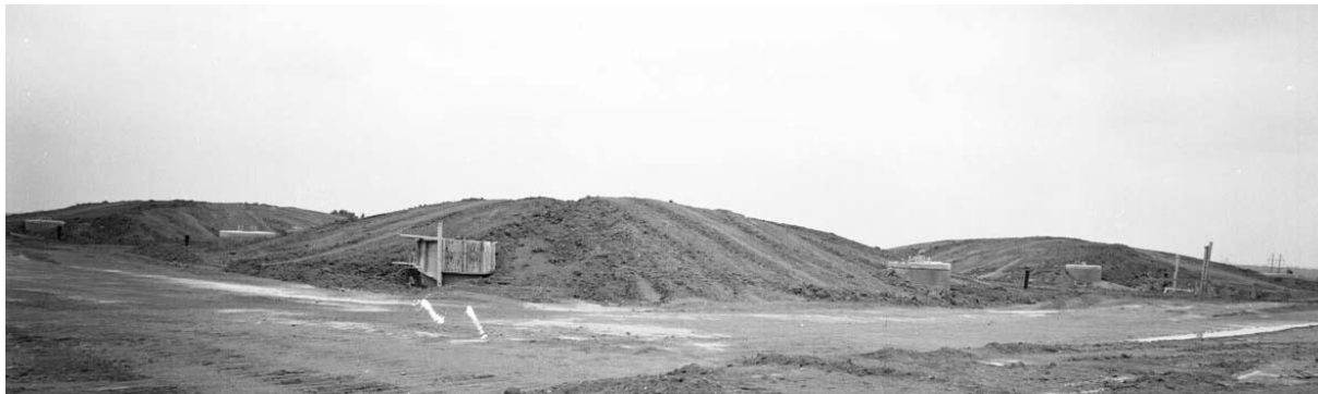
Figure 3.2-53: Type IV Tanks Backfill Complete
