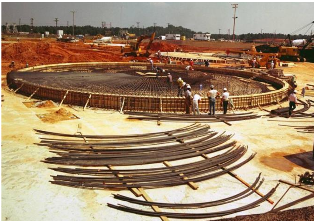
Figure 3.2-29: Early Construction of a Type III and IIIA Tanks Basemat
