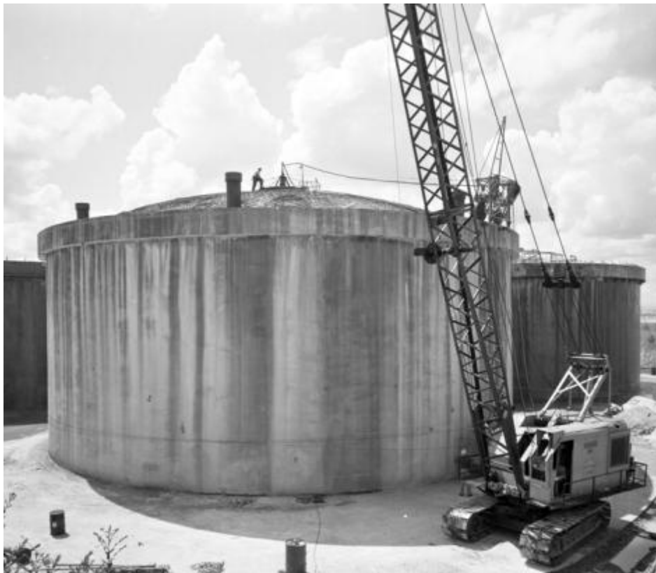
Figure 3.2-49: Type IV Tank Dome Construction
