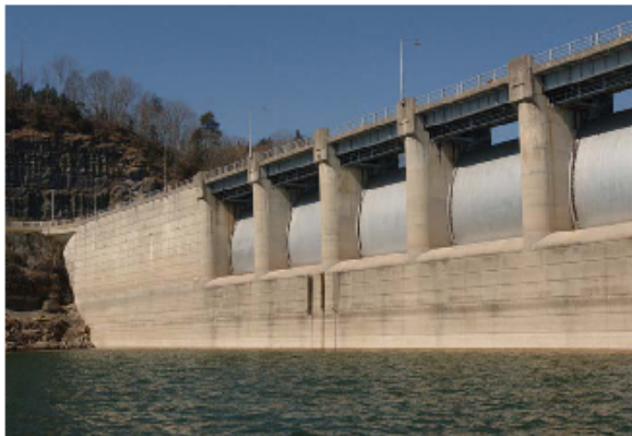
Wolf Creek Dam Spillway
