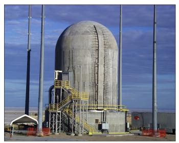
Figure 12.14 Completed pre-stressed concrete containment vessel 1:4 scale model at SNL (Source: Figure 52, NUREG/CR-6906 (SAND2006-2274P)
