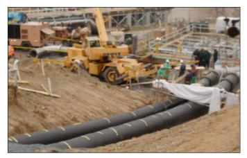
Figure 9.24 Installation of underground Class 3 safety-related HDPE piping
