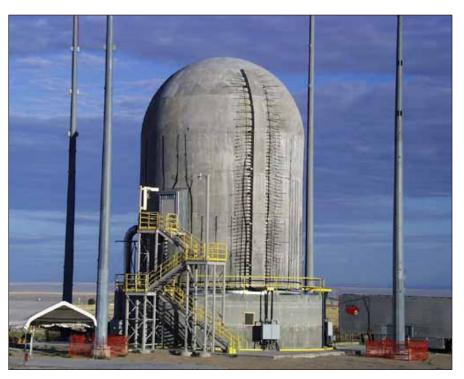
Completed prestressed concrete containment vessel ¼-scale model at Sandia National Laboratories
