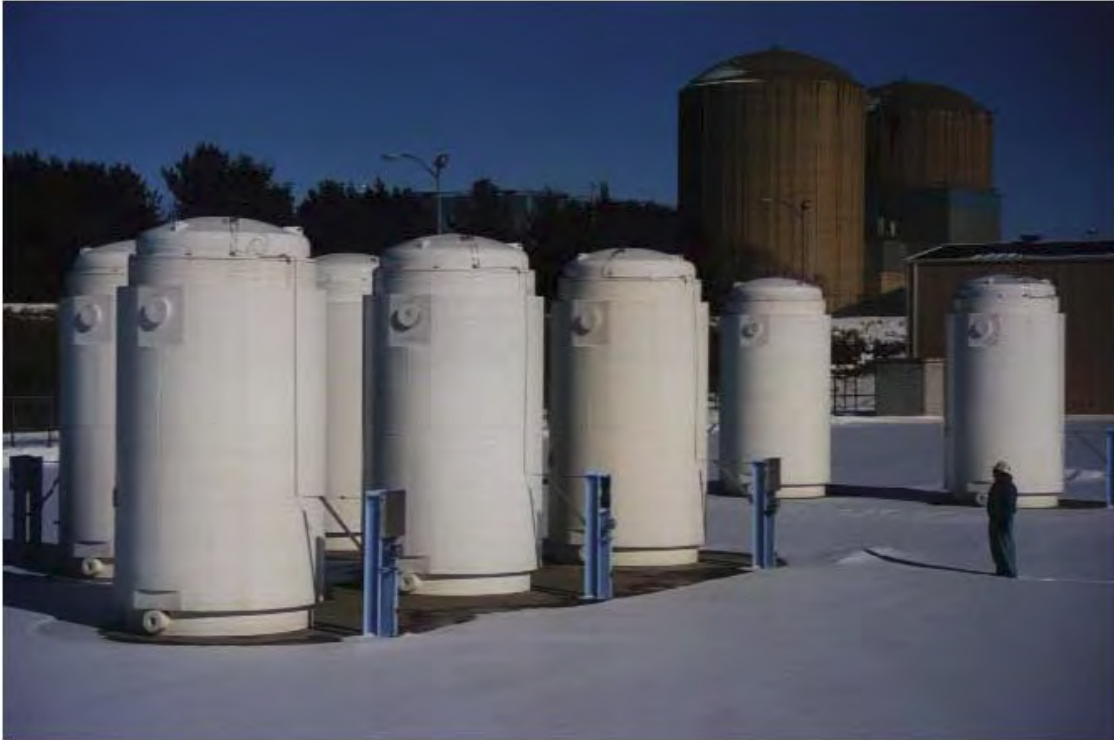
Figure 16-1 Series of Transnuclear (TN)-40 Casks at an Independent Spent Fuel Storage Installation
