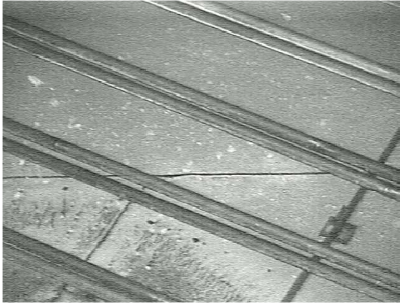
Figure 12. Photograph of the interior of TFF Tank WM-183 after tank cleaning.
