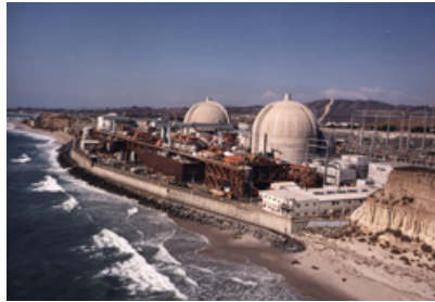
Permanently shutdown reactors at San Onofre Station. Source: NRC.
