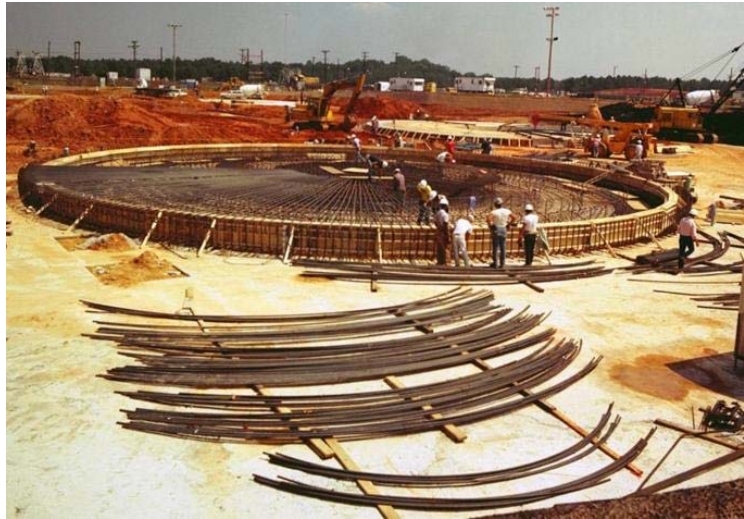
Figure 2.1-44: Typical Type III/IIIA Tank Basemat Construction
