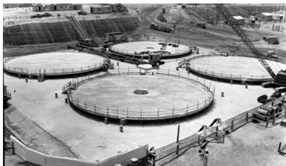
Figure 2.1-36: Type II Tank Basemat Construction
