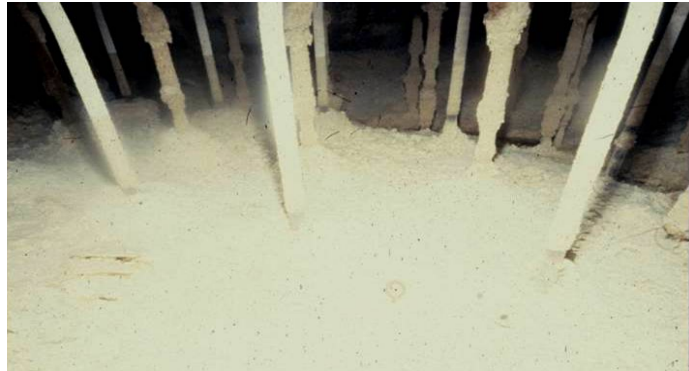
Figure 2.2-1: Saltcake at Bottom of Waste Tank
