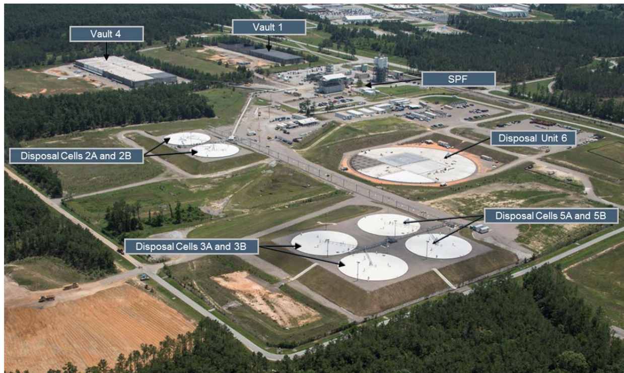
Figure A.3-3: Saltstone Facility (June, 2014)
