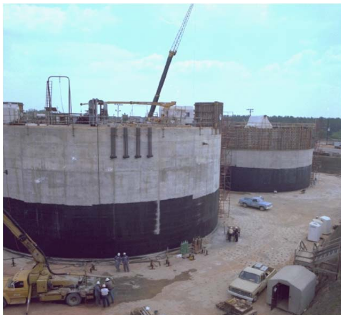
Figure A.2-1: Waste Tanks Under Construction
