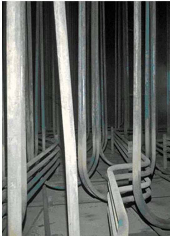
Figure 2.1-40: Typical Type II Tank Cooling Coil Obstacles
