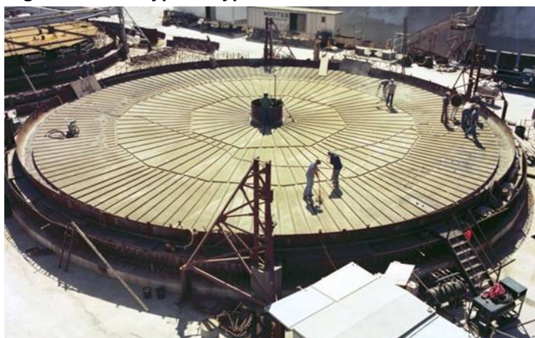
Figure 2.1-46: Typical Type III/IIIA Tank Radial Air Grooves
