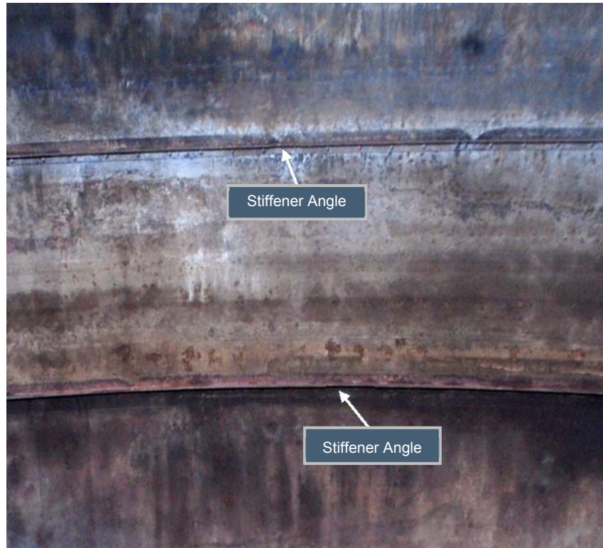
Figure 2.1-52: Typical Type IV Tank Stiffener Angles
