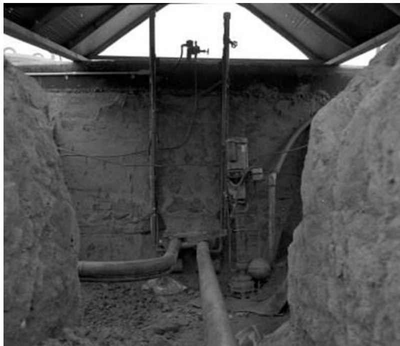
Figure 2.1-57: HTF Waste Tank Transfer Line During Construction
