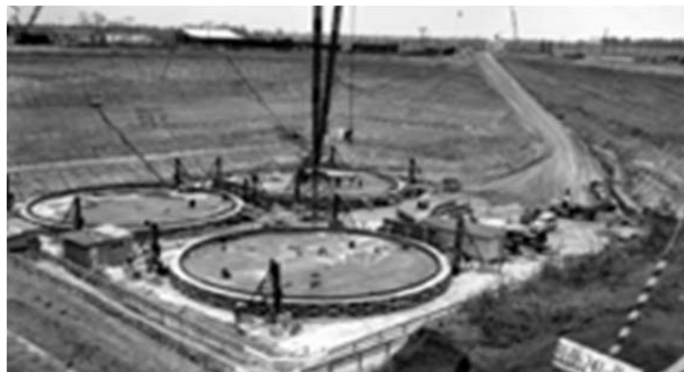
Figure 2.1-30: Type I Tank Basemat Construction
