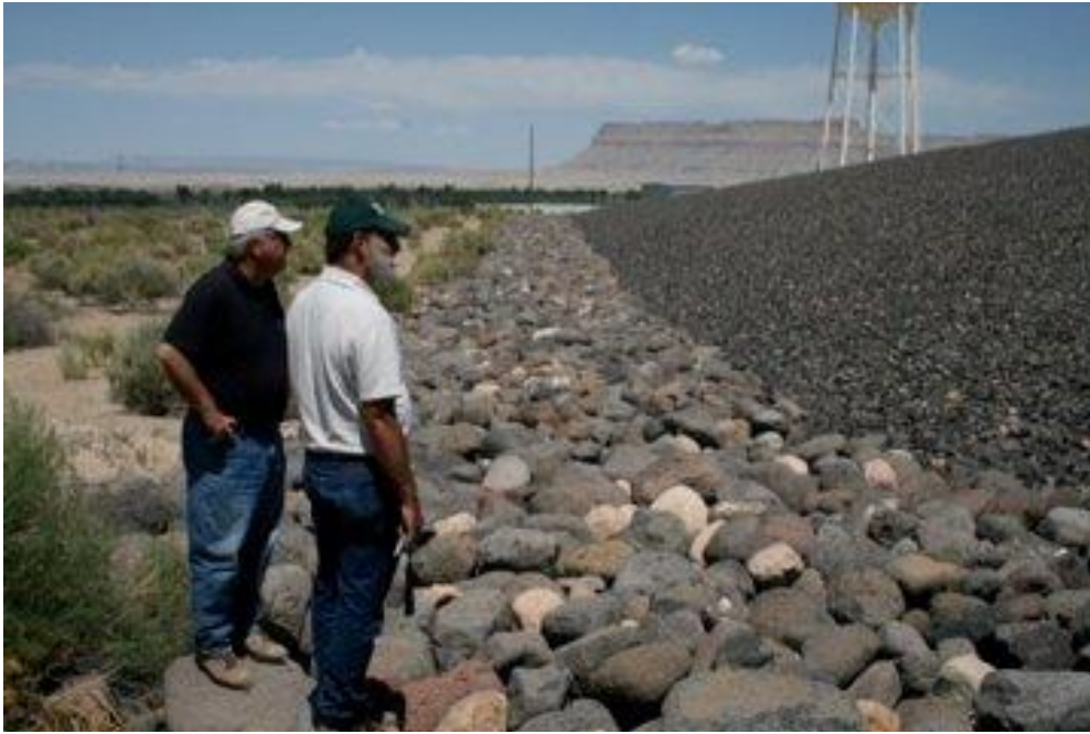
2 3 4 Figure E-8 Example of an Erosion Protection Cover for Uranium Mill Tailings
