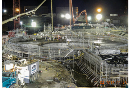
Construction at a nuclear power plant site
