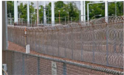
Barriers are part of the physical protection system used at operating reactors to defend against the DBT
