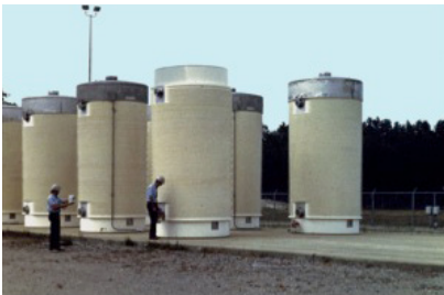
Spent fuel is safely and securely stored in an ISFSI
