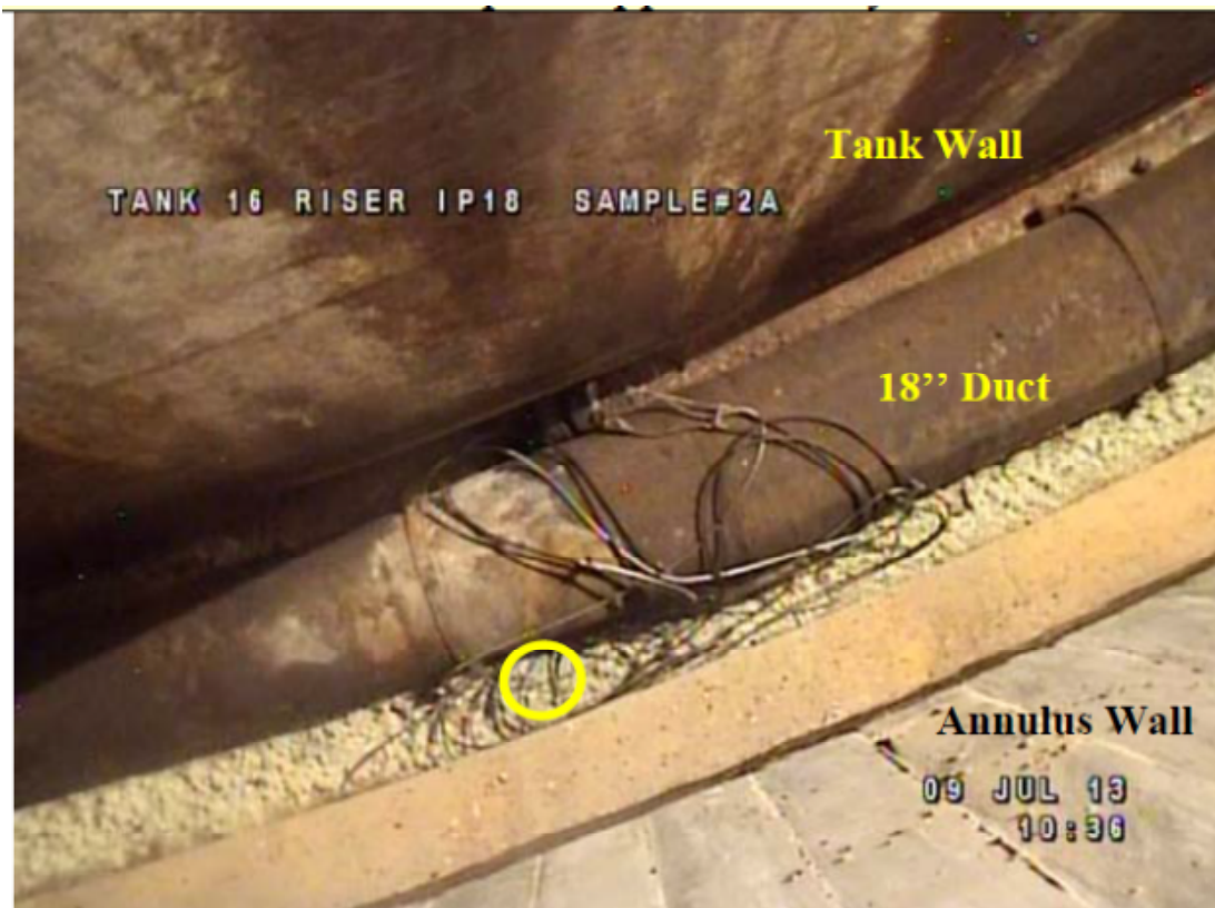
Figure 3 Photograph of Waste Near Sample 2-A (Reproduced from Figure in Section 4.7 of SRR-LWE-2013-00027, page 16).
