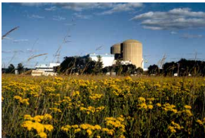
Prairie Island Nuclear Generating Plant, Units 1 and 2
