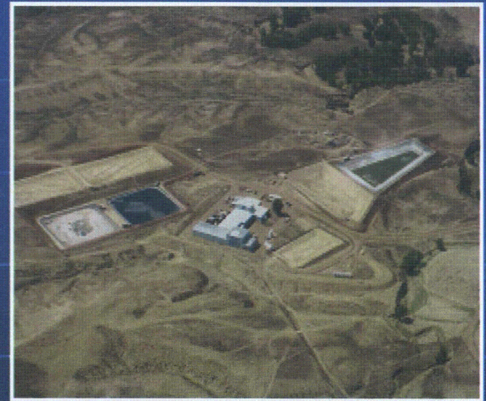
Aerial view of Irigaray processing facility
