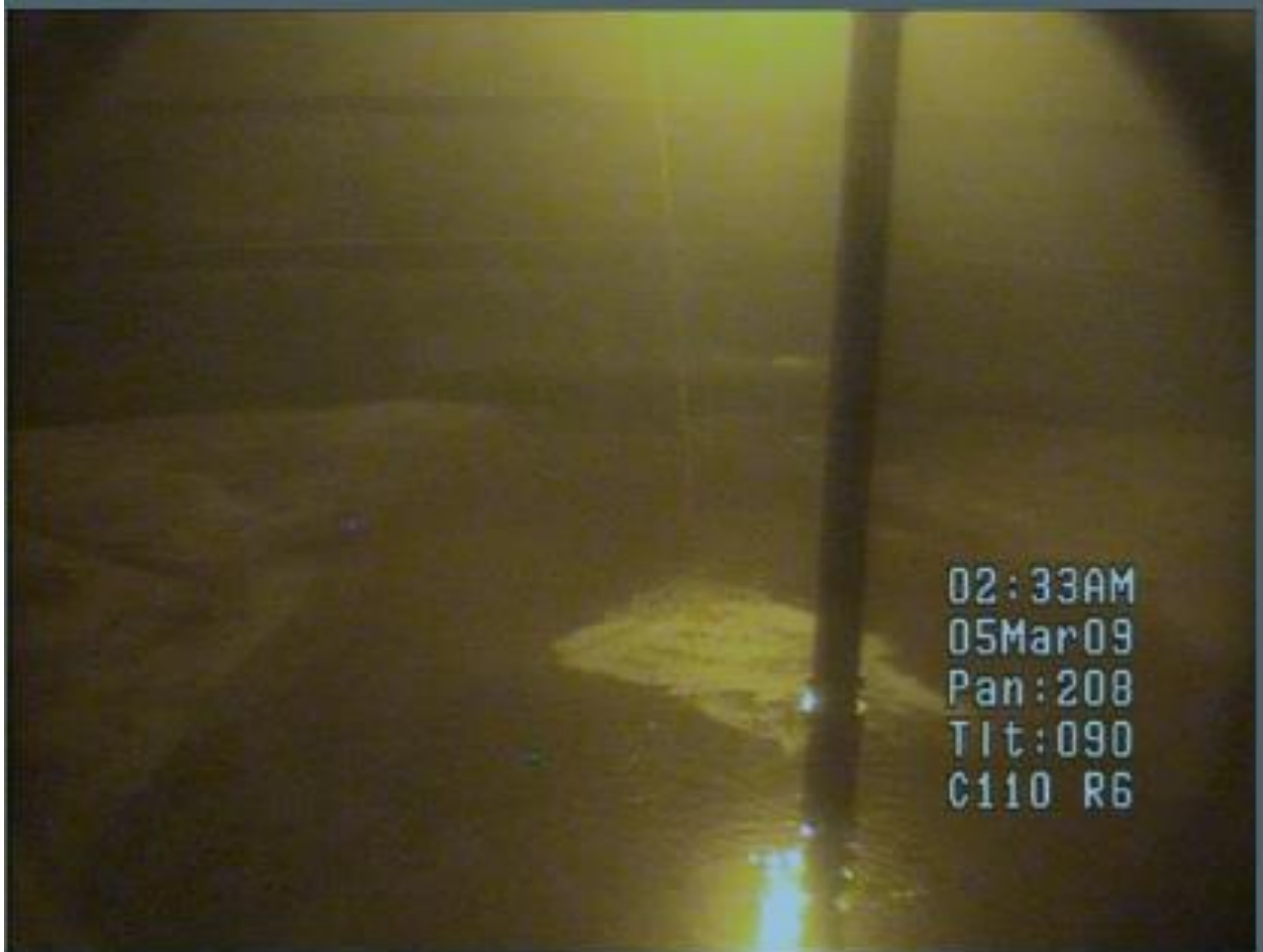
4 Figure 2-18. Tank C-110 Sluicing Photograph.
