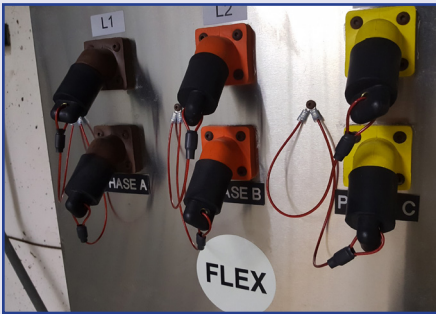
Standard mechanical and electrical connections for the portable equipment were installed at all U.S. plants. (Photo of FLEX Jumper connection panel at St. Lucie nuclear power plant and mechanical connection at Millstone nuclear power plant.)
