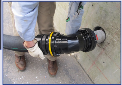
Standard mechanical and electrical connections for the portable equipment were installed at all U.S. plants. (Photo of FLEX Jumper connection panel at St. Lucie nuclear power plant and mechanical connection at Millstone nuclear power plant.)
