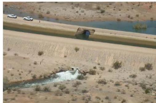
Internal erosion failure through uphill embankment... outflow restricted by culvert. Breach outflow into dry wash.
