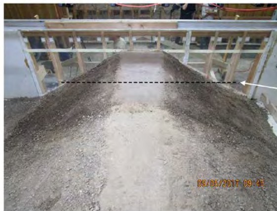
1/2" rebar 18 inches below crest
