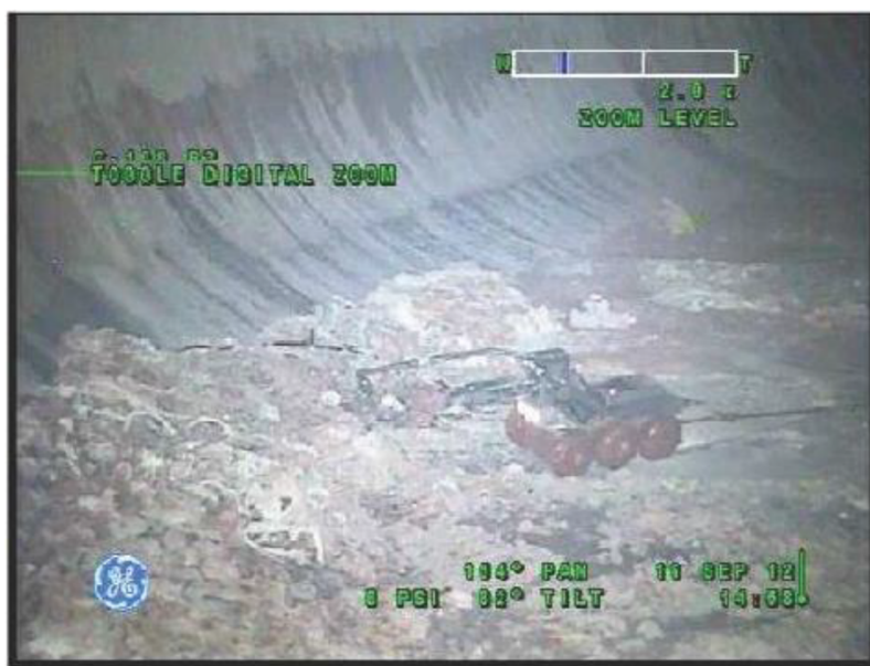
Figure 2-1 Image from Tank C-108 Video Used to Monitor Waste Retrieval
