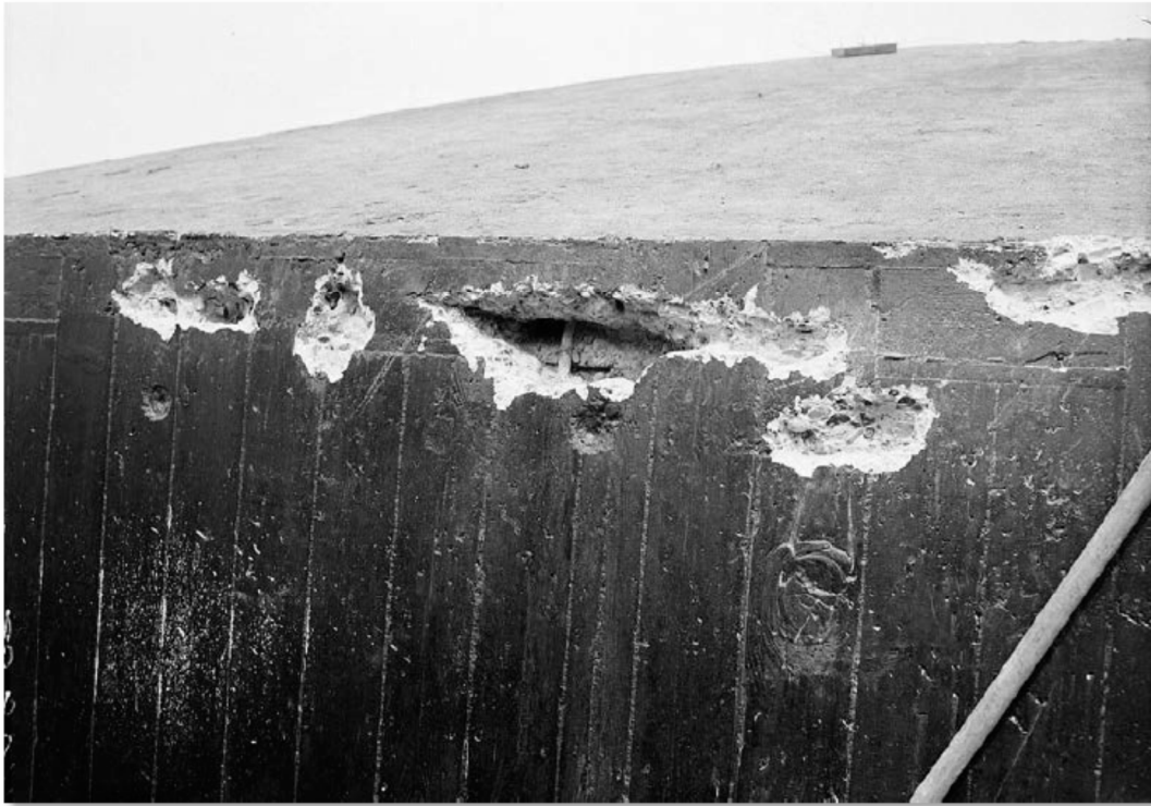
Figure 3-7 Example of Defects in Tank
