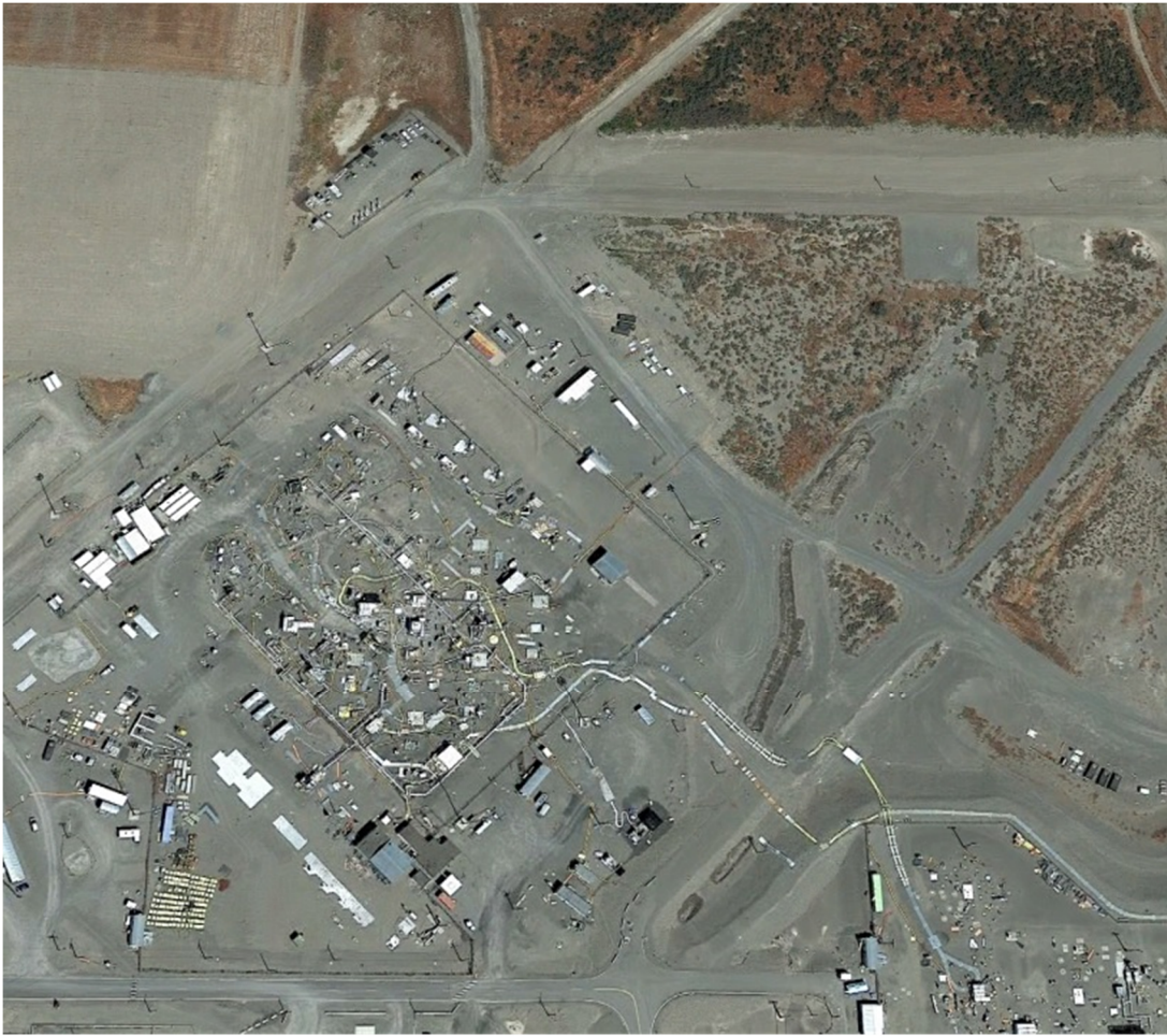
Figure 1-3 WMA C: Buried Single-Shelled Tanks and Ancillary Equipment
