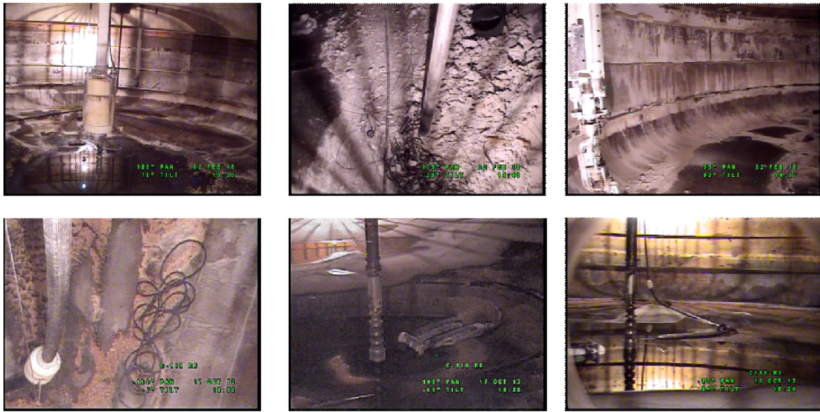
Figure 3-12 Features and Structures Remaining in Waste Tanks
