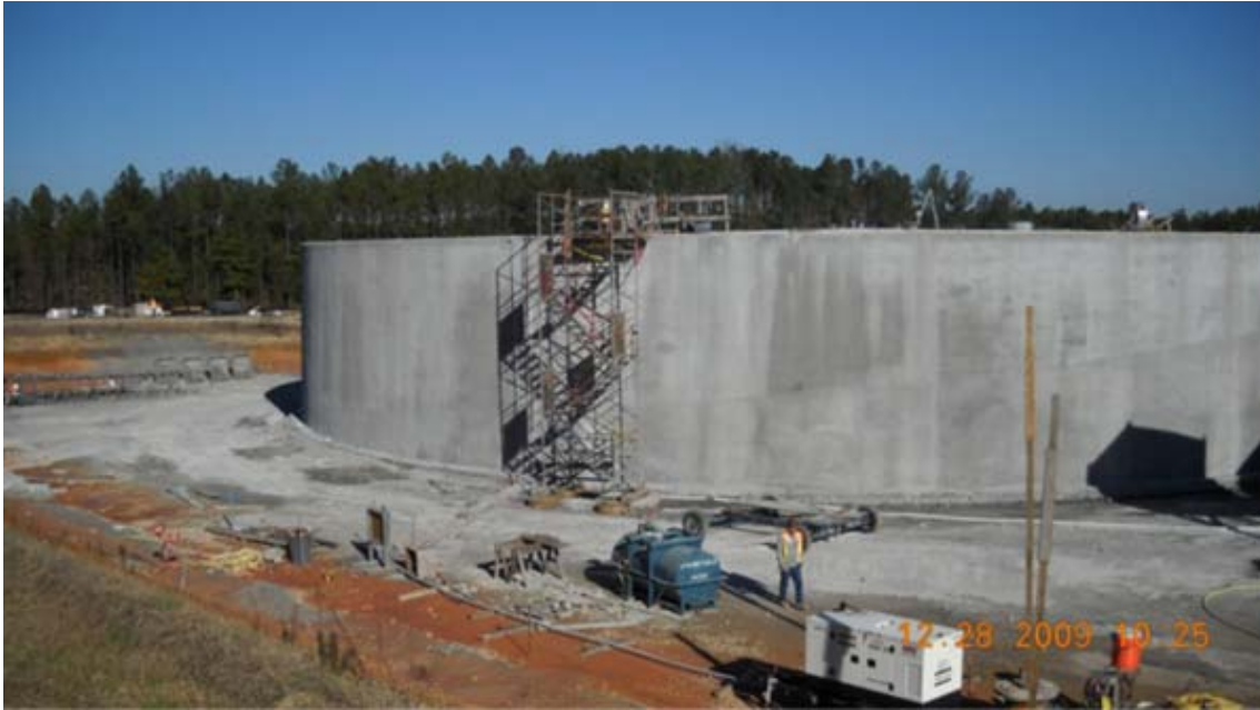
Figure 3.2-13: Typical 150-Foot Diameter SDU Under Construction
