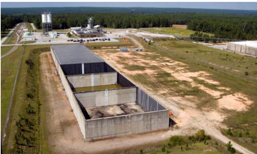
Figure 3.2-3: SDU 1 Exterior View
