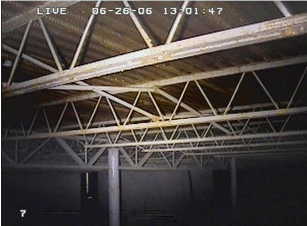
Figure 3.2-12: Interior View of SDU 4 Roof (Cells B through L)
