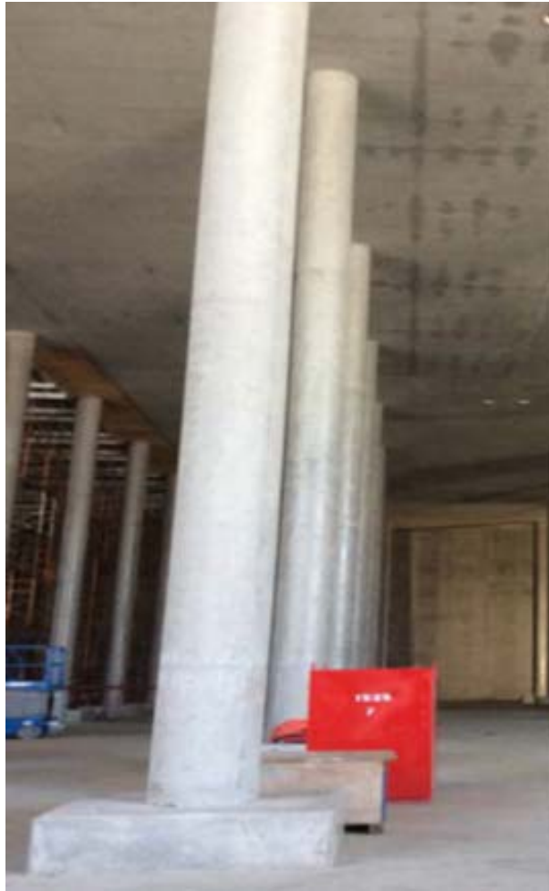
Figure 3.2-27: 375-Foot Diameter SDU Columns as Installed in SDU 6
