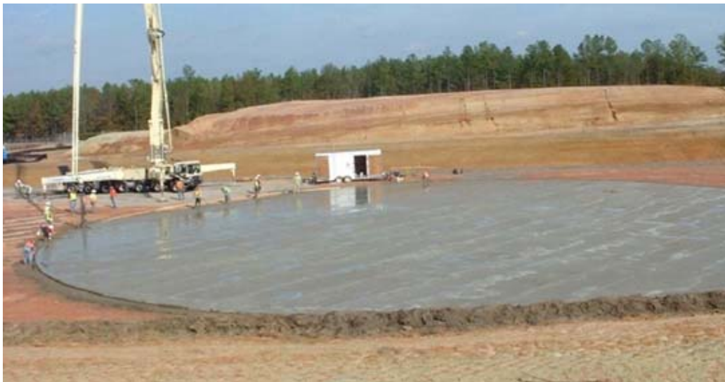
Figure 3.2-20: Placement of Lower Mud Mat for 150-Foot Diameter SDU Construction
