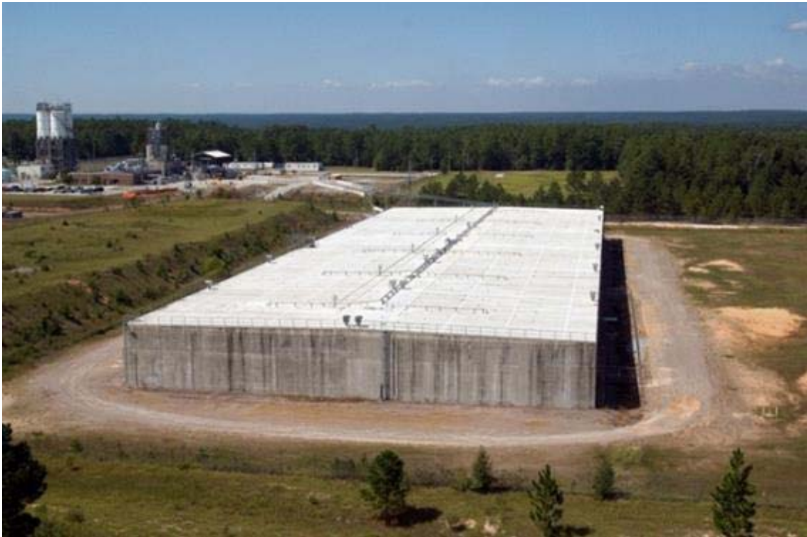
Figure 3.2-7: SDU 4 Exterior View
