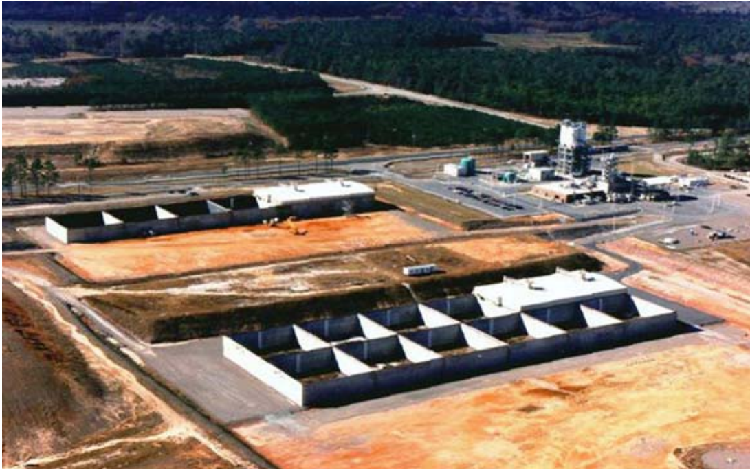
Figure 3.2-2: SDU 1 and SDU 4 Arrangement after Initial Construction
