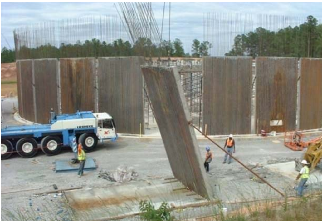
Figure 3.2-18: 150-Foot Diameter SDU Wall Panels Under Construction
