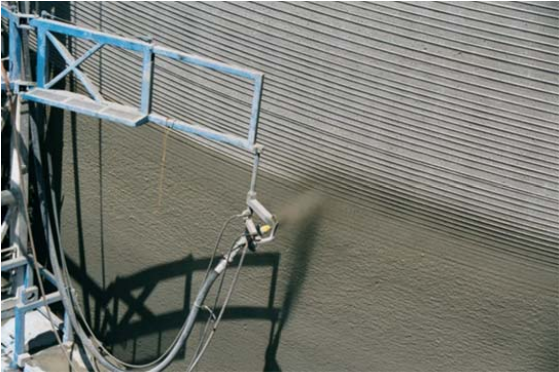
Figure 3.2-26: 375-Foot Diameter SDU with Pre-Stress Wire Wrapping Covered with Shotcrete
