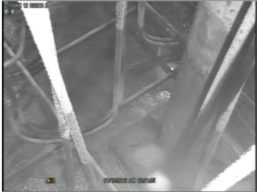
Figure 1. Residual WIR on the Floor of the Tank 12H Primary Appears Similar to Mud Cracks. Light Reflects off a Pool of Water beyond the Column in the Bottom Image. Date of Video: January 19, 2016.
