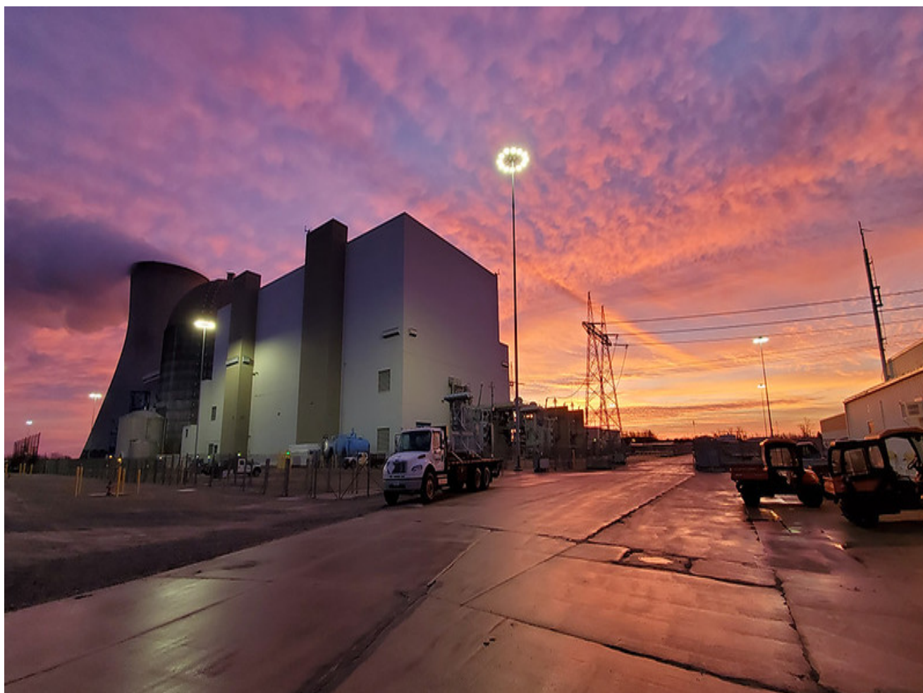
Callaway Nuclear Generating Station
