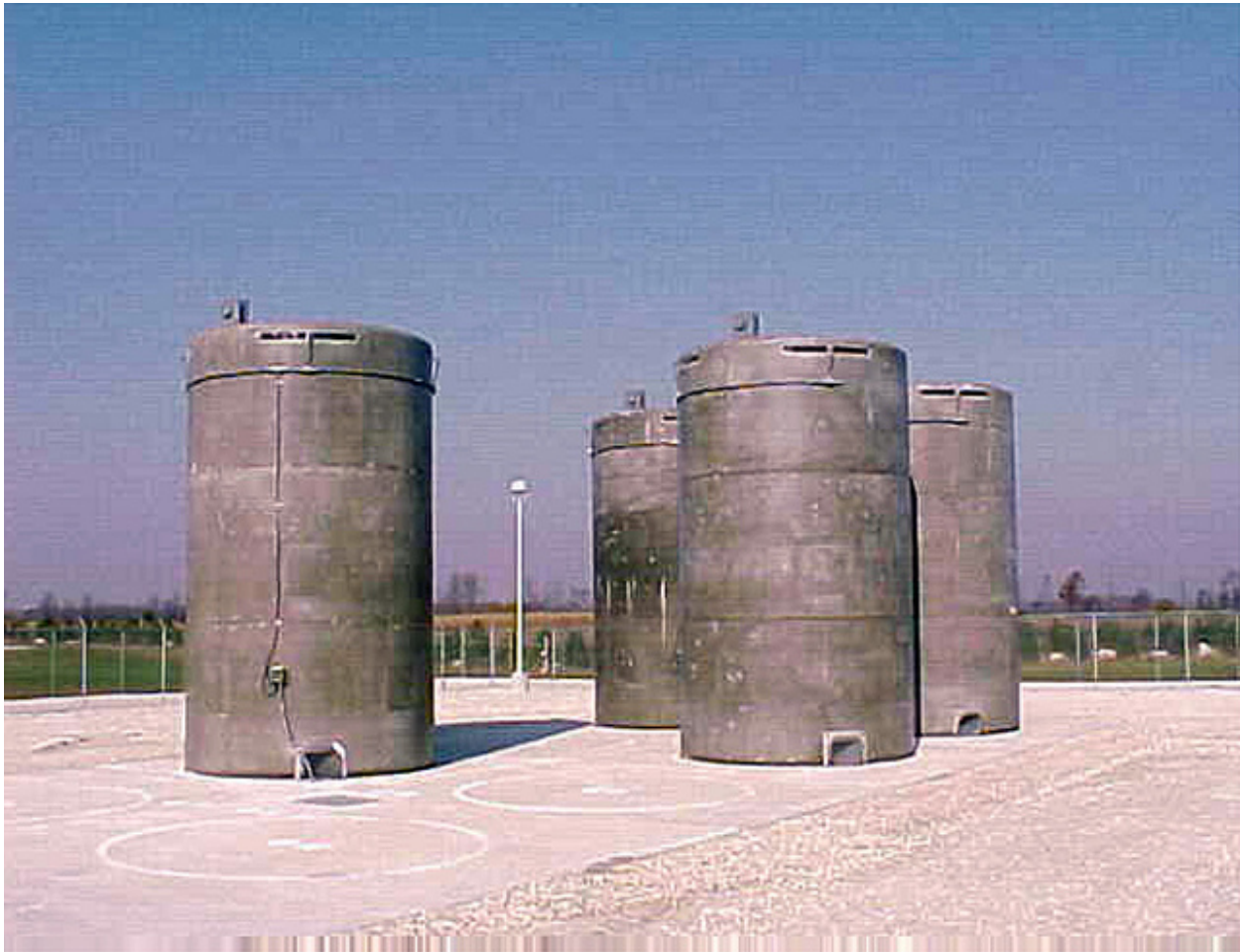
Spent Fuel Dry Cask Storage
