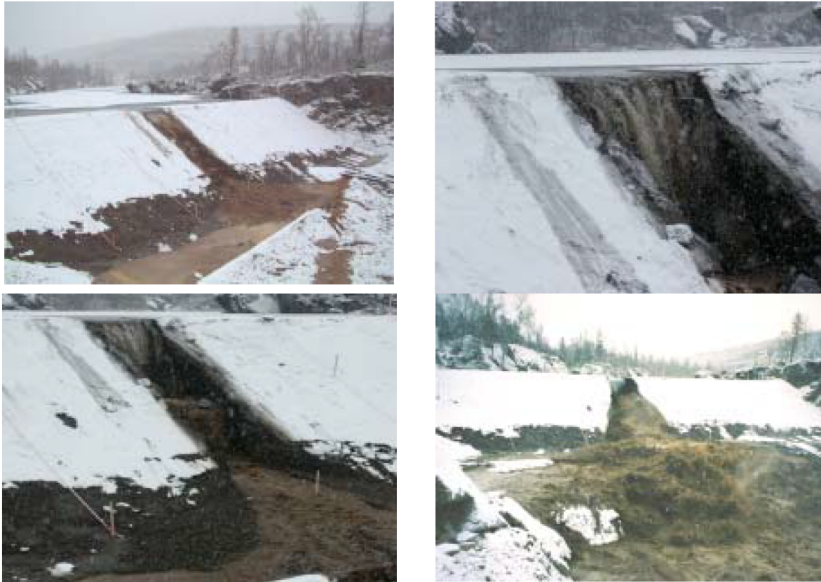
Figure 6-2 Headcut development during IMPACT test of homogeneous gravel dam, 2-2002 (from IMPACT WP2 Technical Report: Section 4).
