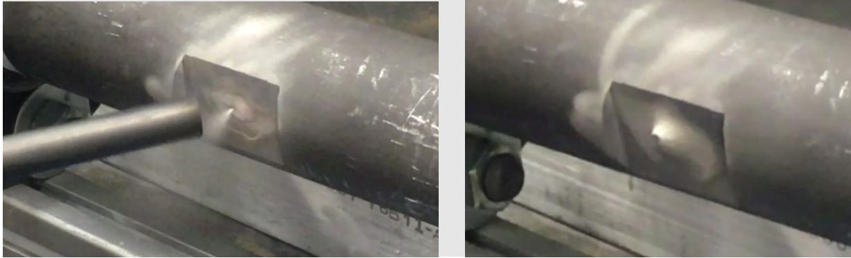
Figure 3-8 Repair of active leak using CS by VRC Metal Systems. Left: water leak; right: final repair. Pressure of the pipe was ~100 psi during and 1,000 psi after the repair (Ross and Alabi 2019).
