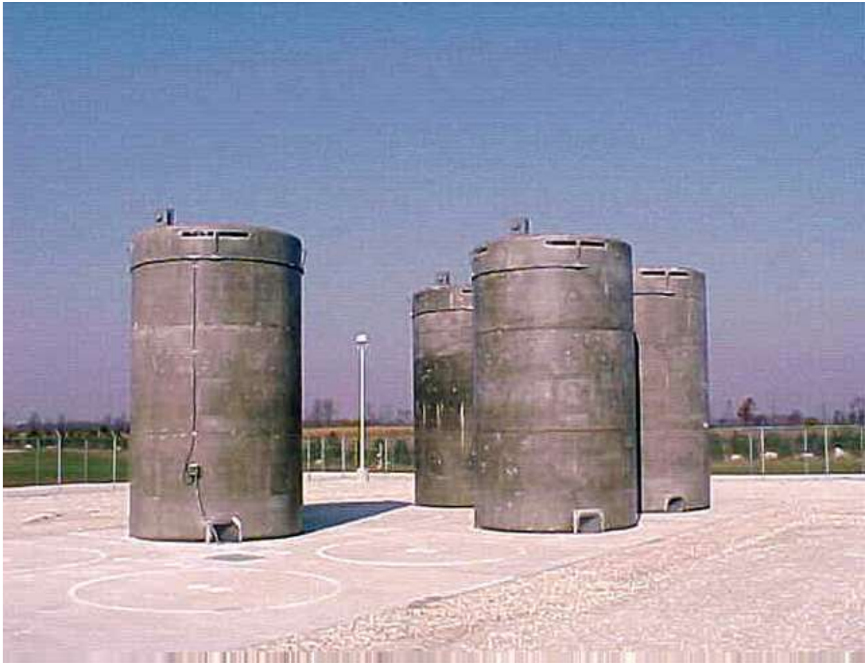
Spent Fuel Dry Cask Storage
