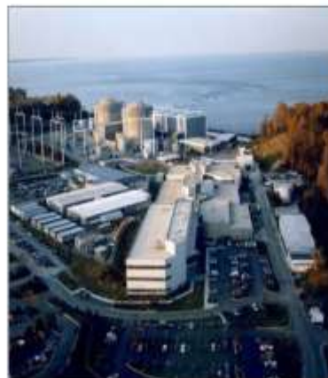
Calvert Cliffs Nuclear Power Plant, Lusby, MD
