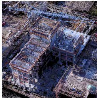
Reality Capture (drone+laser scanner)
