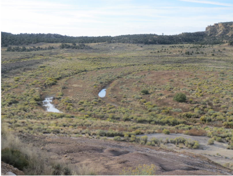
Figure 4: Ponding on the existing disposal cell cover at the Church Rock Site after a rainfall event in 2015.
