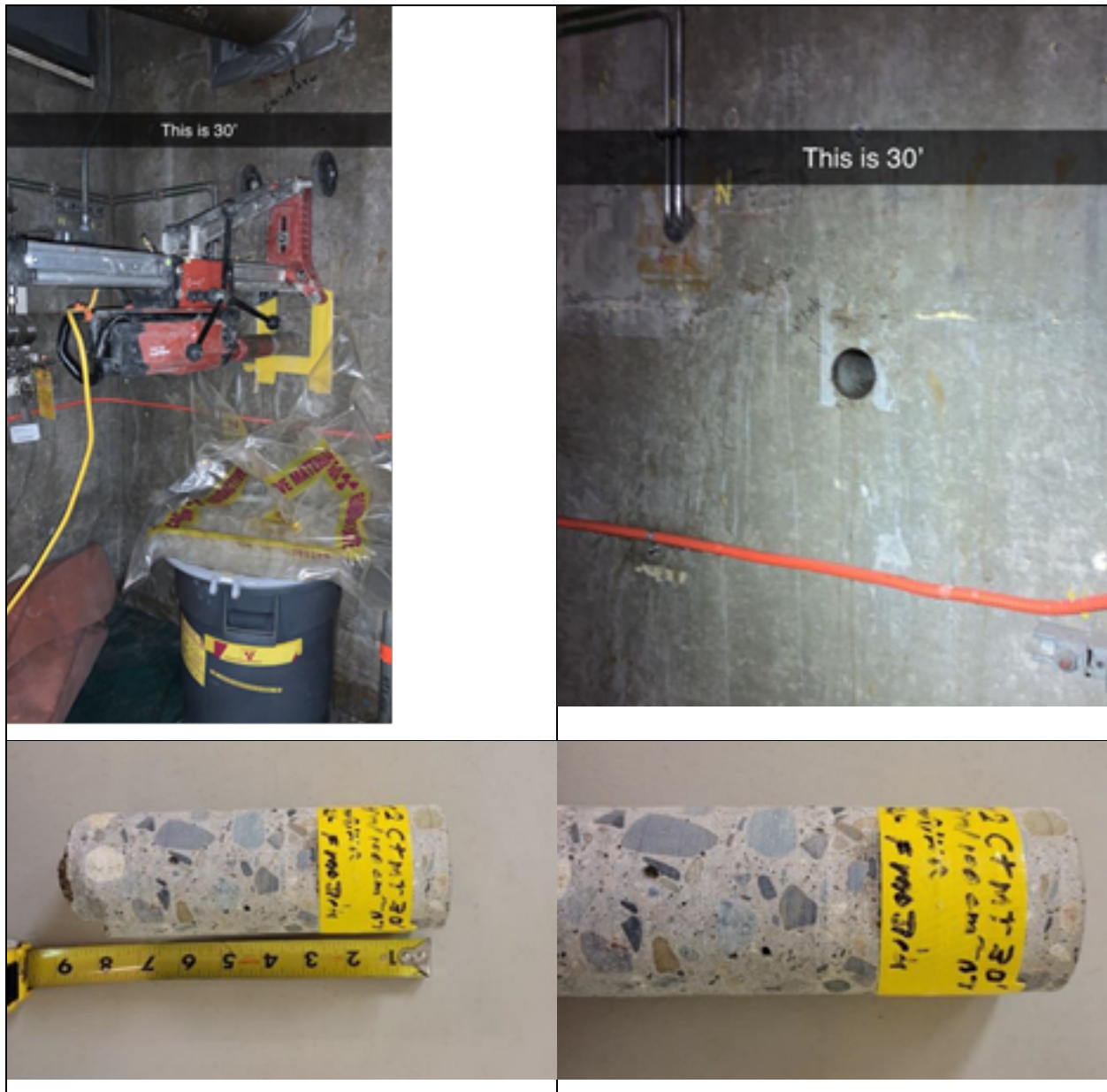
Figure 3-2 Cored specimen at 30 ft elevation
