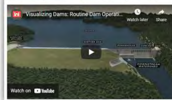
Visualizing Dams - Routine Dam Operations
