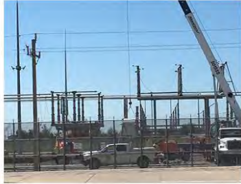
Restoration of DAEC Off Site Power
