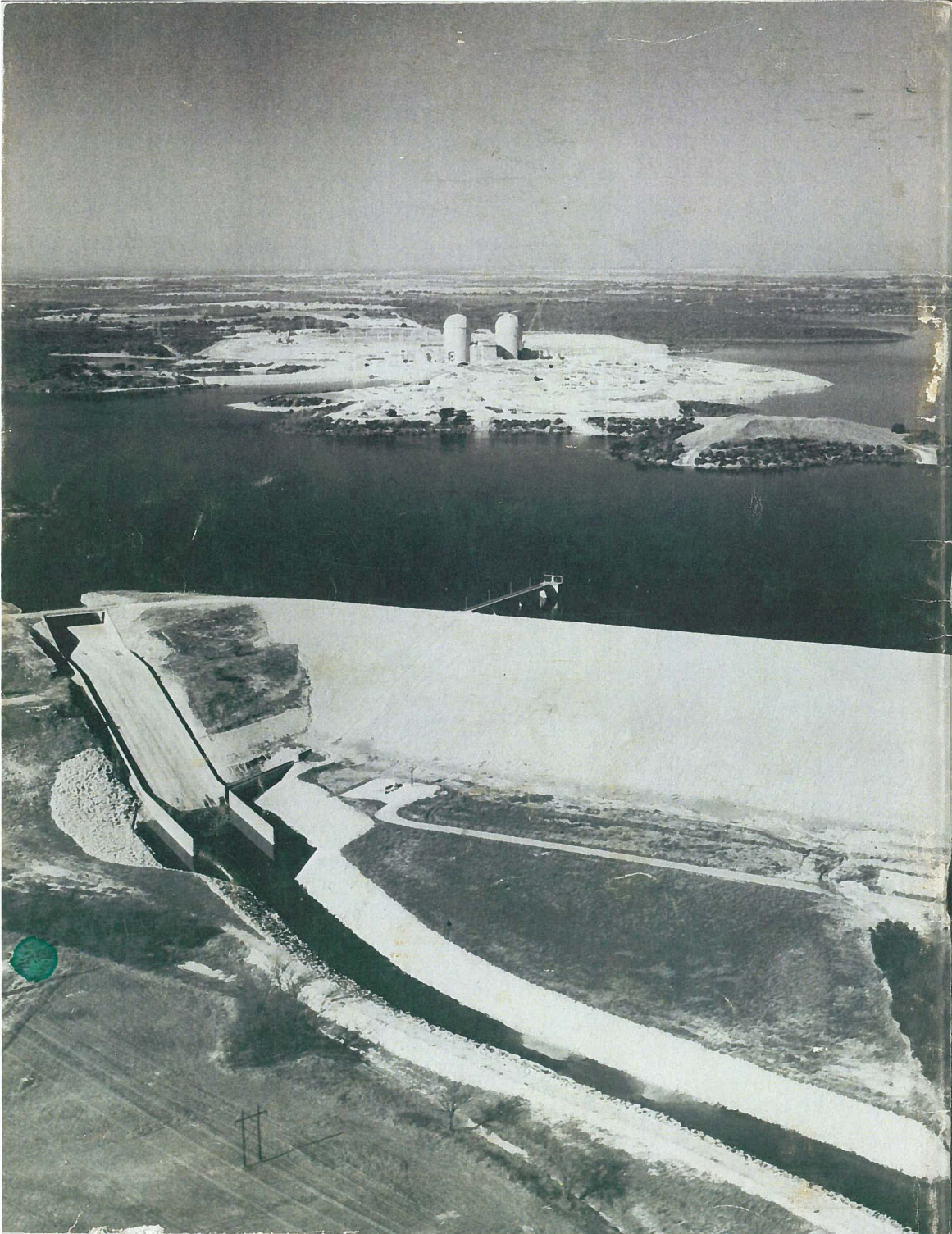
Figure 3.8-10 Late-Construction Photograph of CPNPP Showing Structures, Buildings, SCR, Dam and Spillway, Facing West-Northwest
