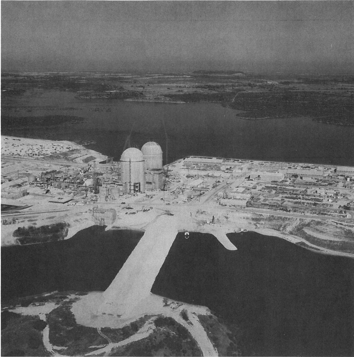
Figure 3.8-8 Late-Construction Photograph of CPNPP Showing Structures, Buildings, and SCR, Facing North
