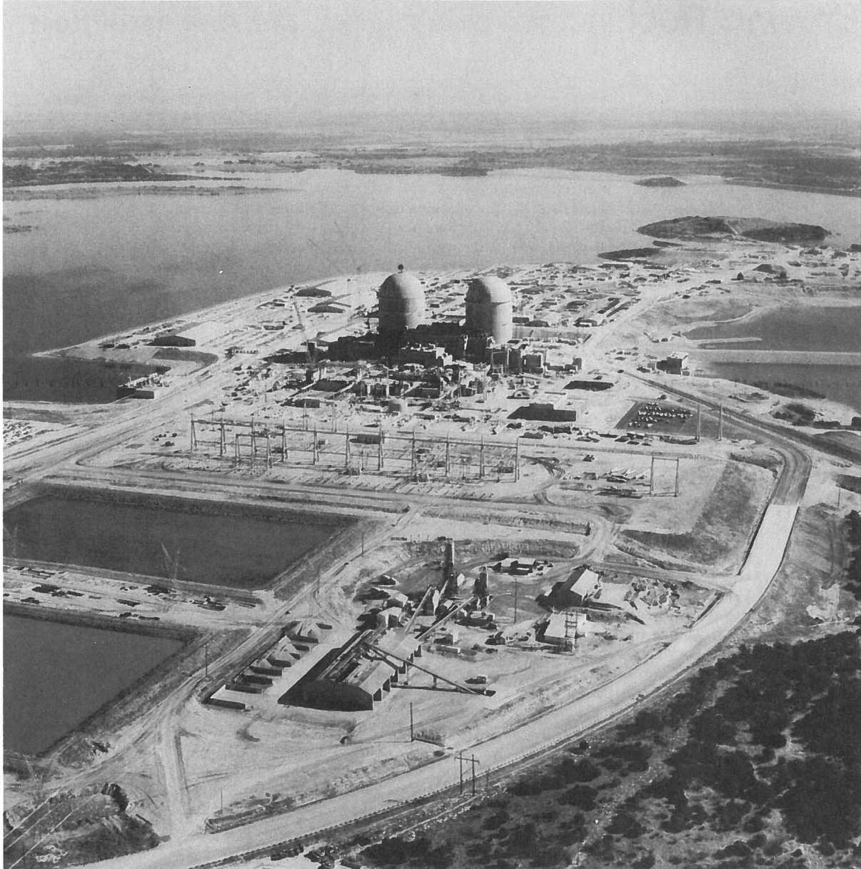
Figure 3.8-9 Late-Construction Photograph of CPNPP Showing Structures, Buildings, and SCR, Facing Northeast
