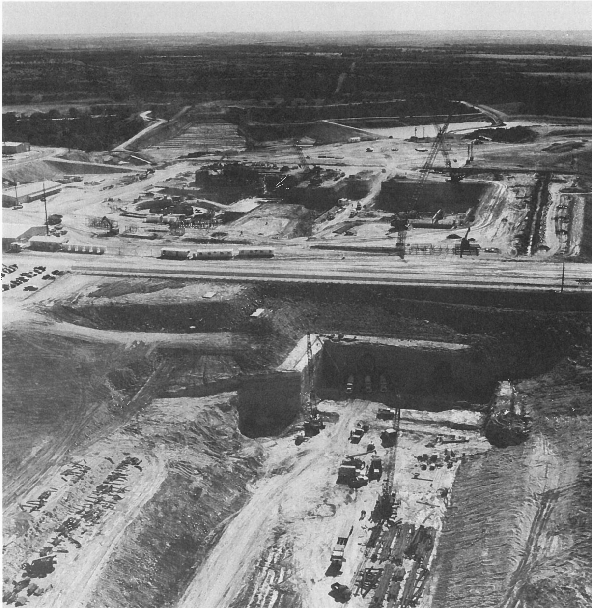
Figure 3.8-7 Construction Photograph of CPNPP Showing Areas Excavated for Structures, Facing South
