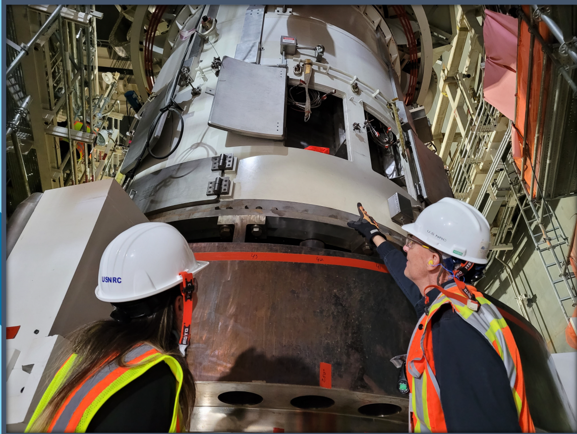
Senior Resident Inspector Brian Kemker and Joylynn Quinones-Navarro viewing the Uni 3 reactor vessel integrated head package.
