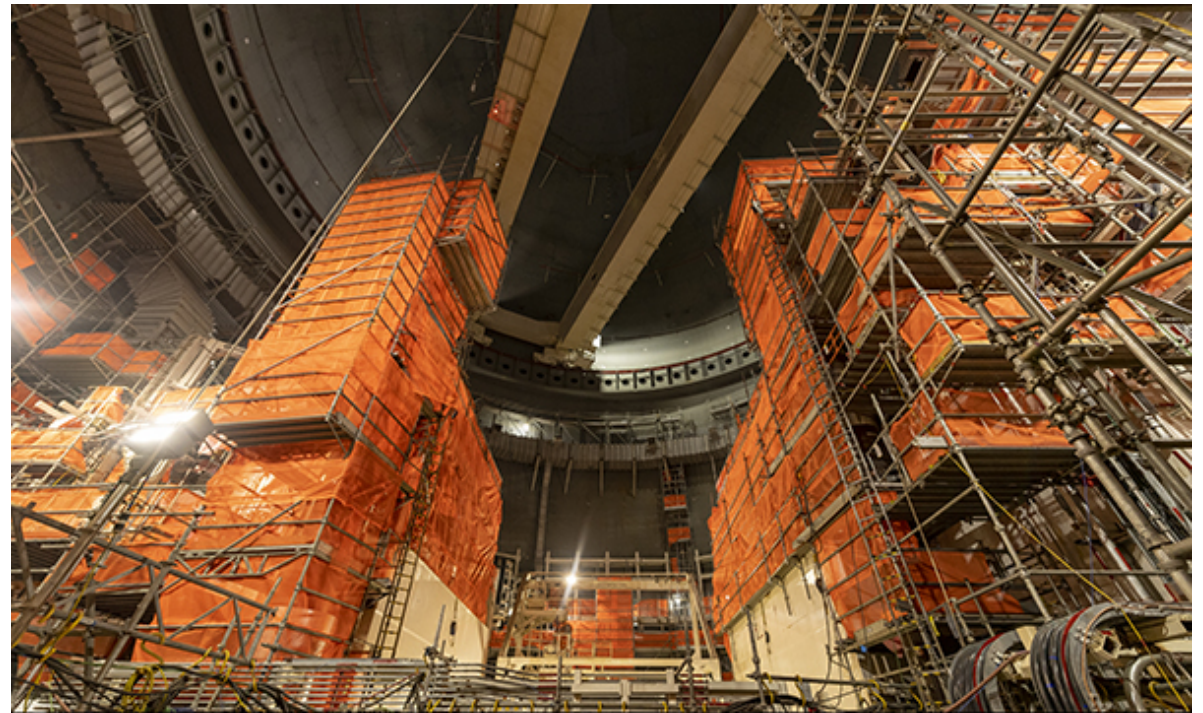
Vogtle Unit 4 Containment
