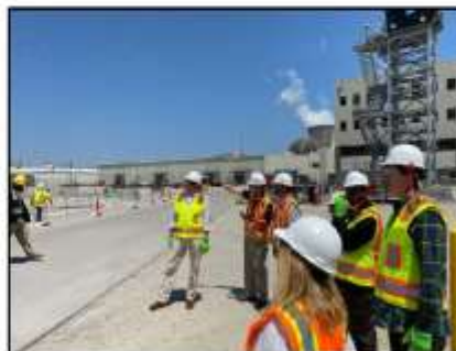
NRC OIG team tours the Vogtle Units 3 and 4 construction project, Waynesboro, Georgia (Image: OIG, with permission)
