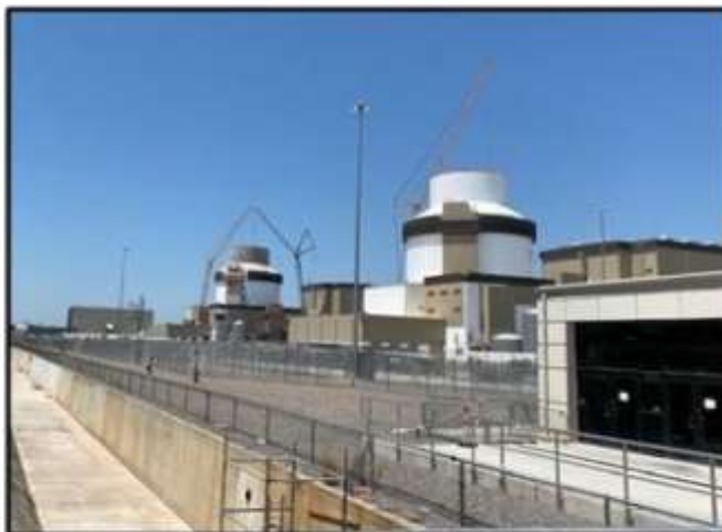
Vogtle Units 3 and 4 Under Construction (Source: NRC OIG, used with permission)
