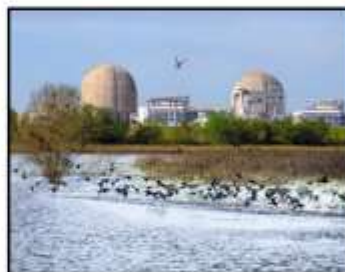
South Texas Project, Units 1 and 2, Bay City, Texas (Photo courtesy of © STP)
