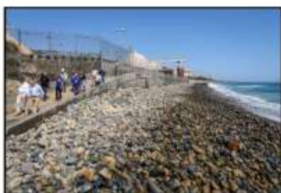
NRC OIG team tours the seawall at the decommissioning San Onofre Nuclear Generating Station, San Clemente, California (Image: OIG, with permission)
