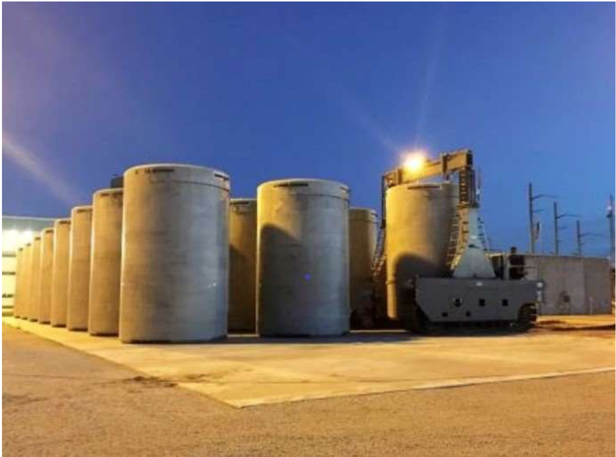
Spent Fuel Dry Cask Storage
