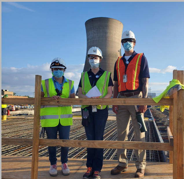
NRC inspectors (left to right) Katherine Warner, Liz Andrews and Mark Henrion observe workers preparing and pouring concrete for a dry cask storage pad on the Three Mile Island plant site in Pennsylvania.
