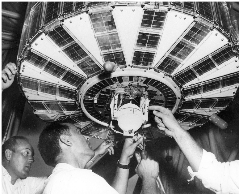
Figure 2-4 Installation of the SNAP generator on a Transit satellite
