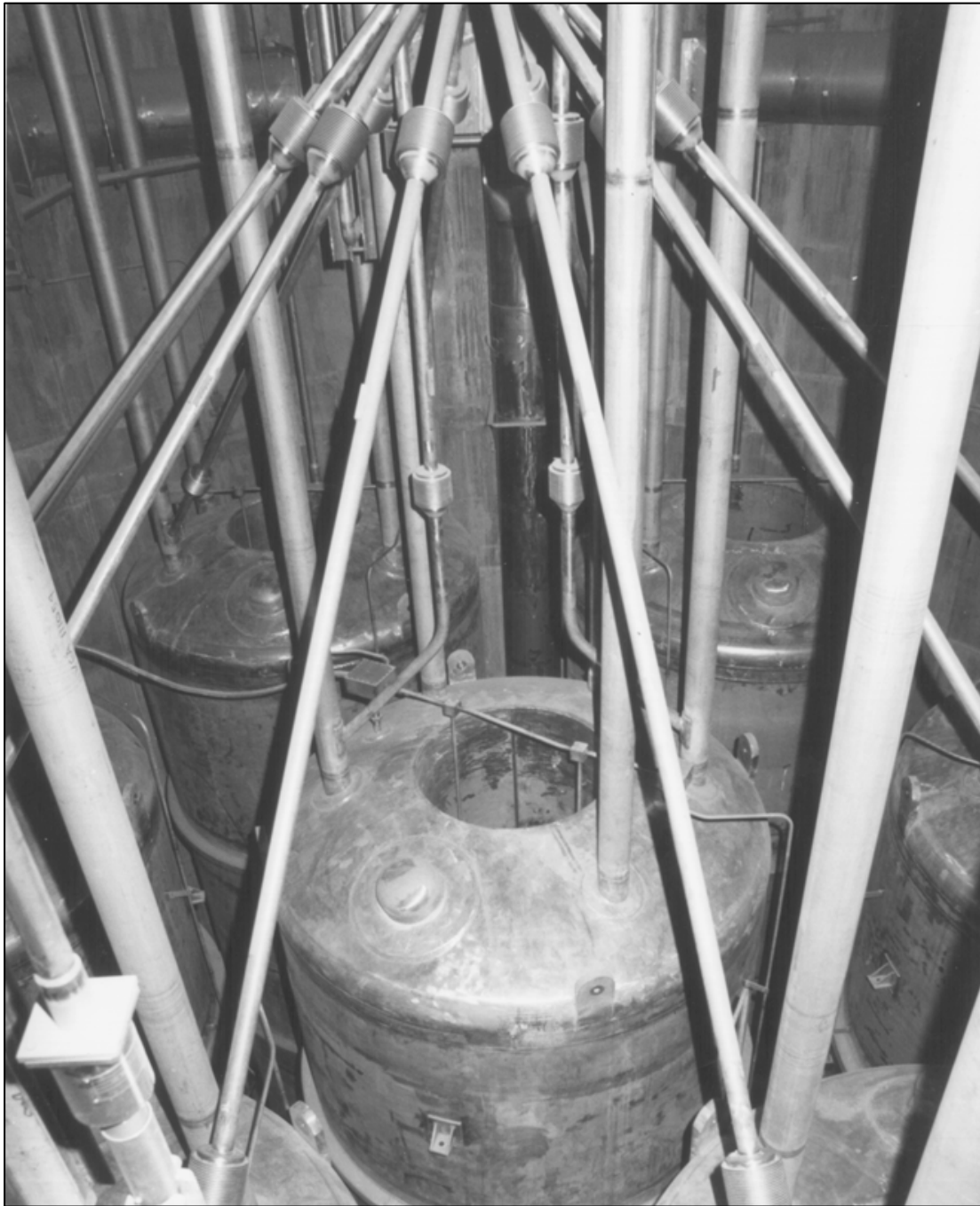
Figure 2-41. Historical photograph of sloped bin fill piping, vertical retrieval piping, and annular bins in Calcined Solids Storage Facility 6 (EDMS ID 7188224).
