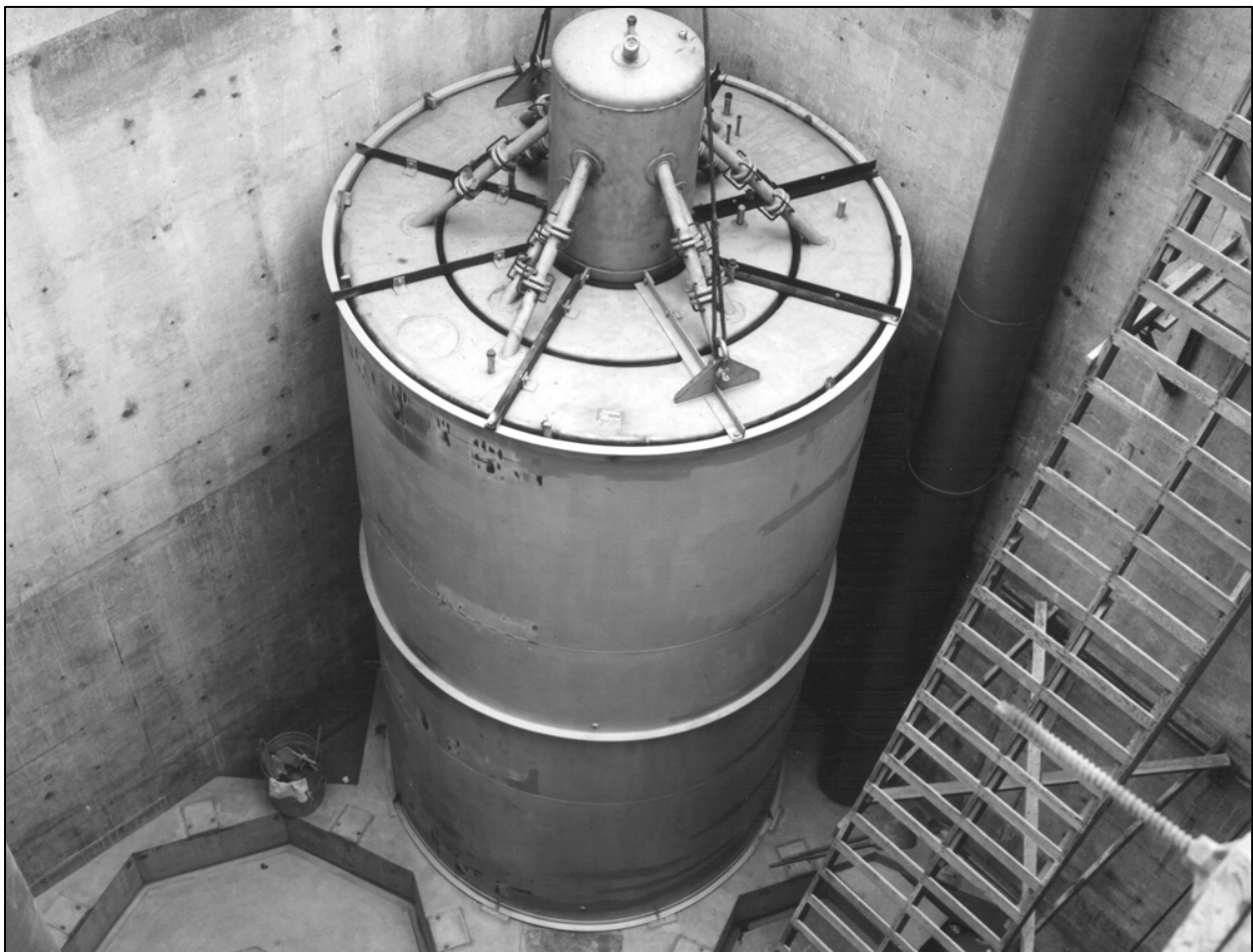
Figure 2-31. Historical photograph of VES-WCS-115-2 placed in the Calcined Solids Storage Facility 1 storage vault (EDMS ID 7188225).
