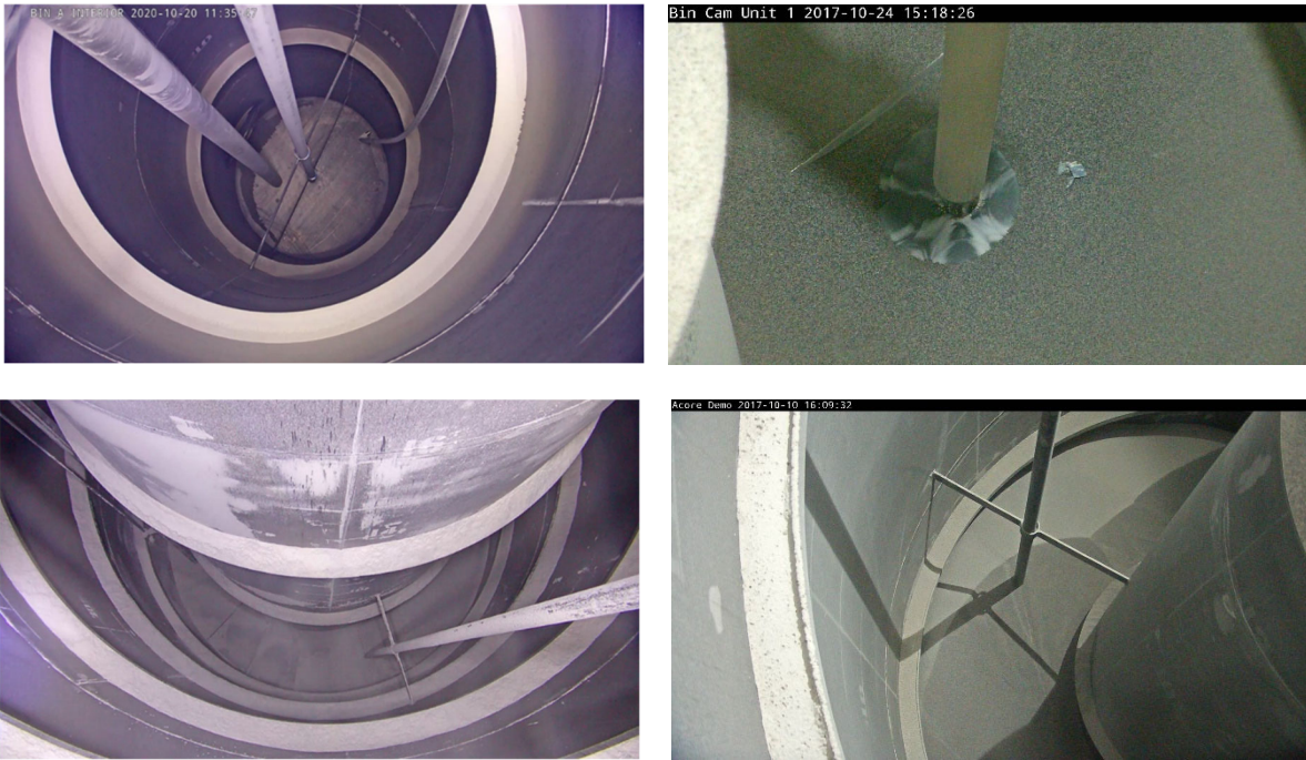
Figure 5-10. Video monitoring system images from inside Calcined Solids Storage Facility 1 during technology testing.
