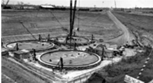
Figure 2.1-30: Type I Tank Basemat Construction
