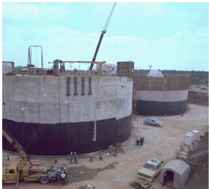
Figure A.2-1: Waste Tanks Under Construction
