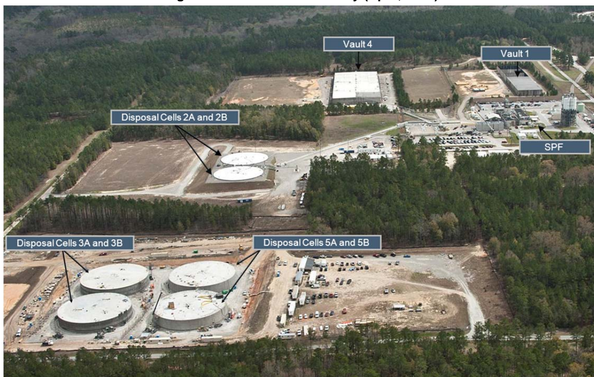
Figure A.3-3: Saltstone Facility (April, 2012)
