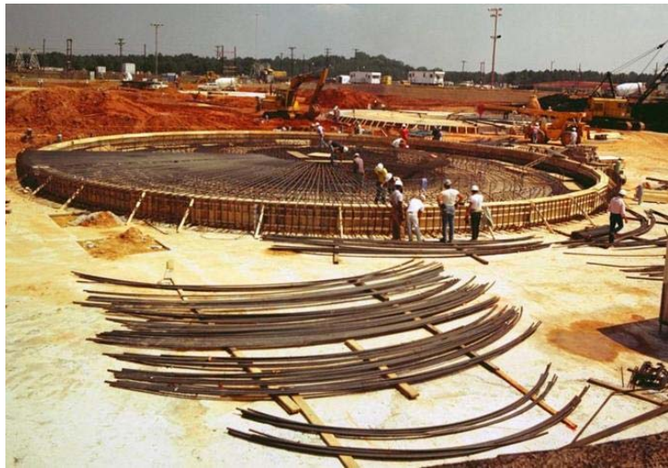
Figure 2.1-44: Typical Type III/IIIA Tank Basemat Construction
