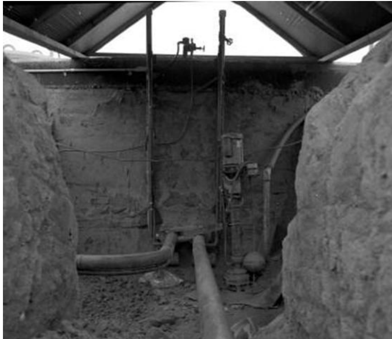
Figure 2.1-57: HTF Waste Tank Transfer Line During Construction
