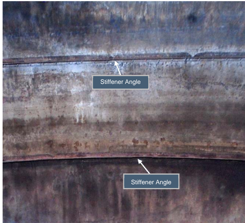
Figure 2.1-52: Typical Type IV Tank Stiffener Angles
