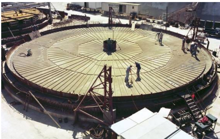
Figure 2.1-46: Typical Type III/IIIA Tank Radial Air Grooves
