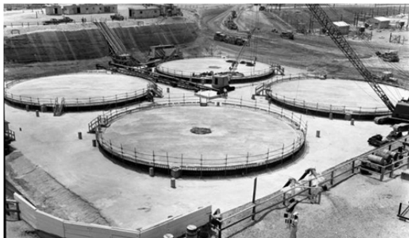
Figure 2.1-36: Type II Tank Basemat Construction
