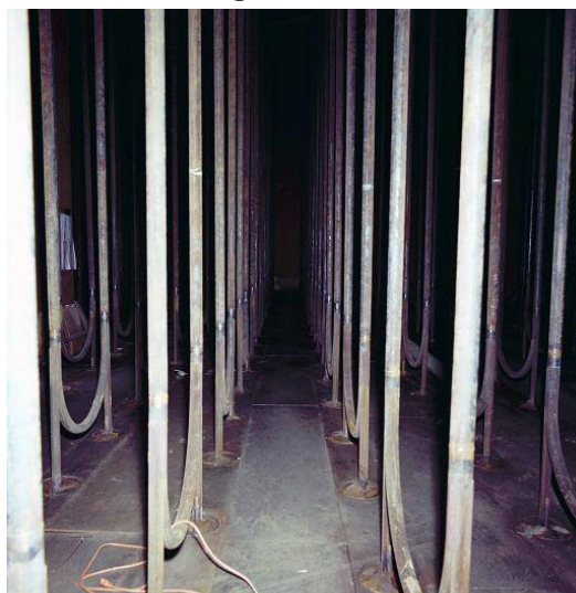
Figure 2.1-48: Typical Type IIIA Tank Cooling Coils During Construction
